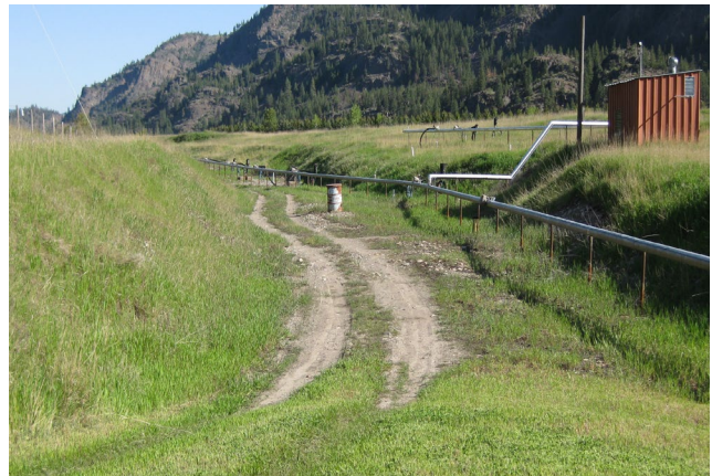
Surface impoundment after sludge removal
