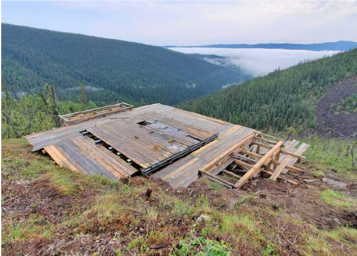
Figure 4. Wooden drill site platform.
