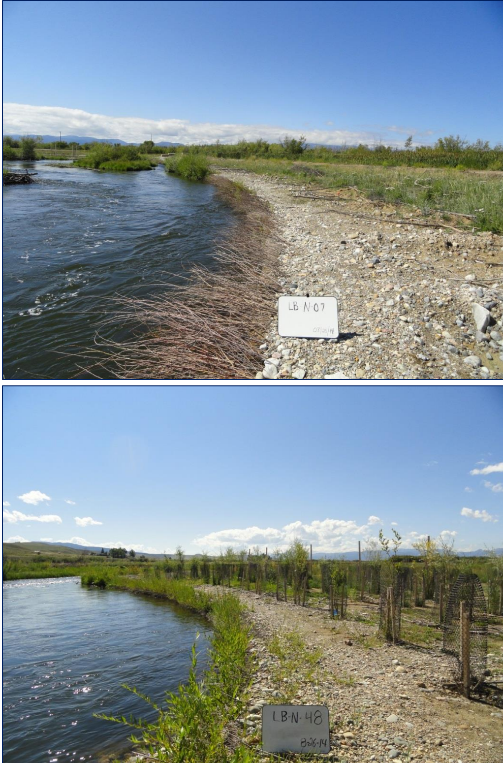
Figure 5-9. Example double vegetated soil lift streambank treatments with relatively low (2%; upper panel) and relatively high (40%; lower panel) woody canopy cover in Phase 1 of Reach A of the Clark Fork River Operable Unit, 2014.
