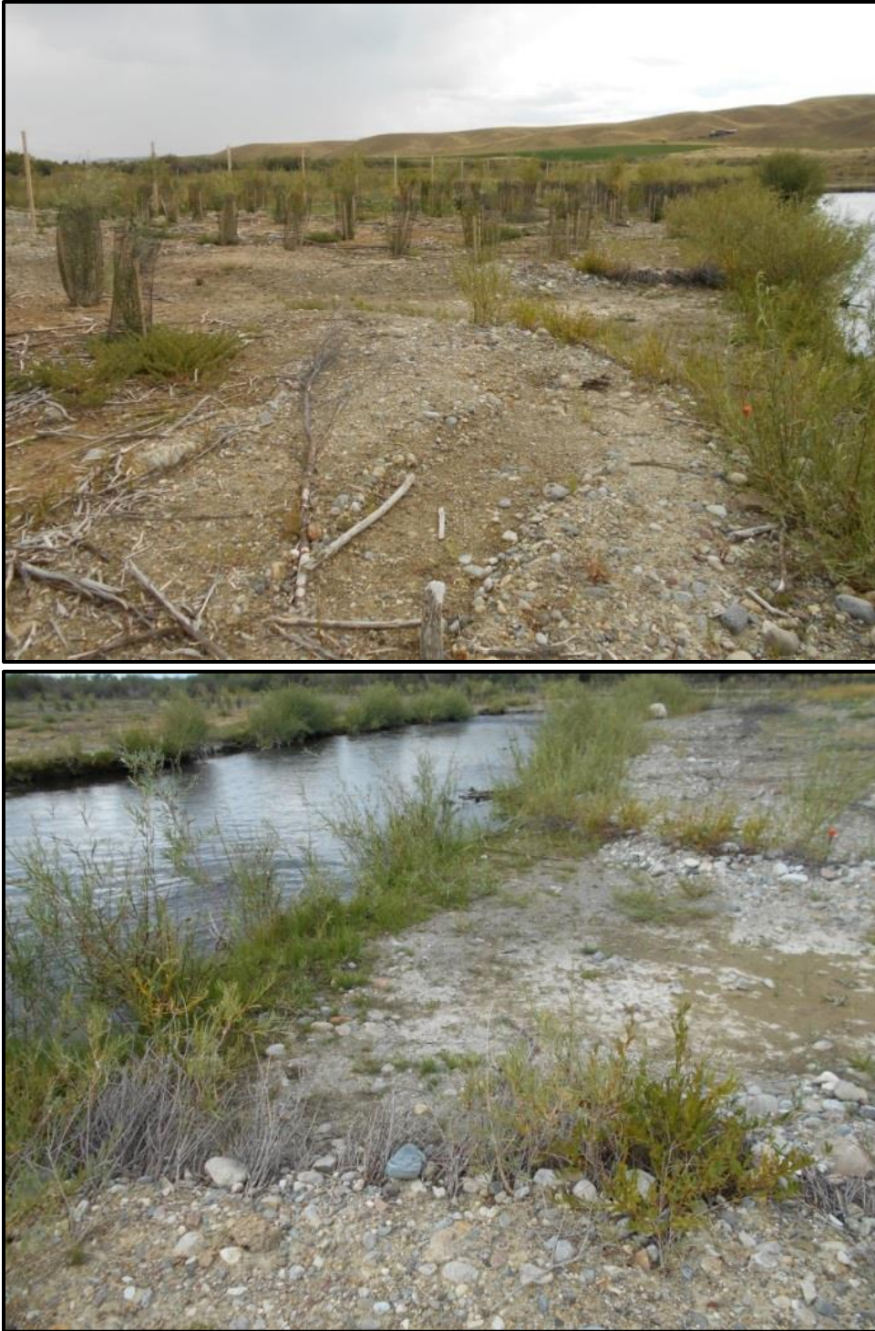
Figure 4-13. Views of designed secondary channel inlet in Phase 1 of the Clark Fork River Operable Unit on August 20, 2014. Mean daily streamflow at the Clark Fork River at Galen site [USGS, 2015b] was 100 cfs on August 20, 2014.
