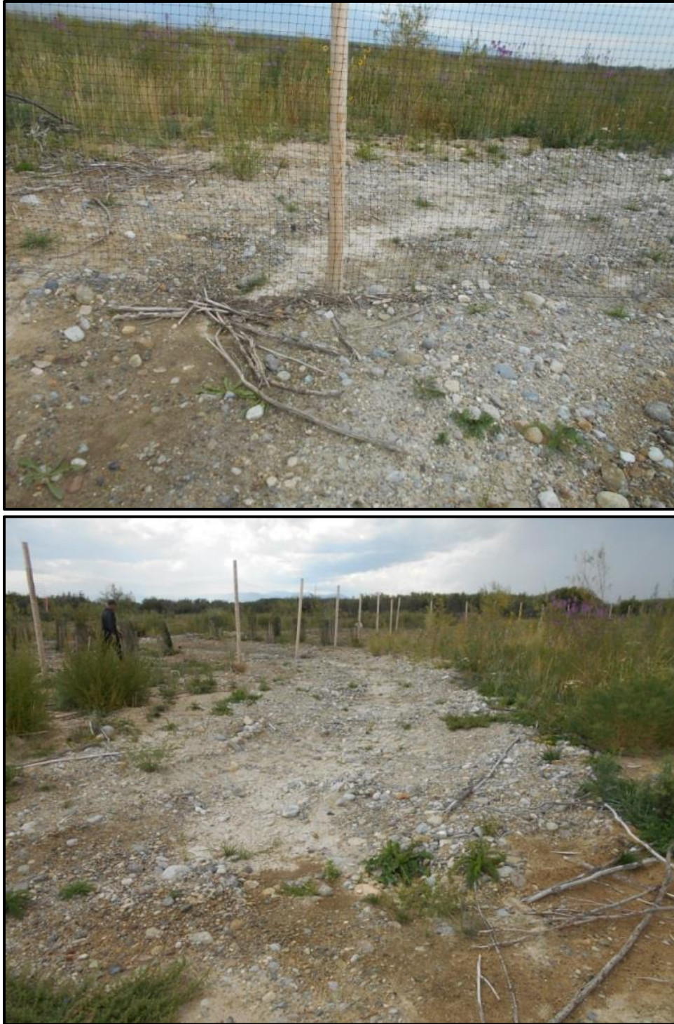
Figure 4-15. View of designed secondary channel where the channel passes through browse protection fence (upper panel) and after passing through the fence (lower panel) in Phase 1 of the Clark Fork River Operable Unit on August 20, 2014. Mean daily streamflow at the Clark Fork River at Galen site [USGS, 2015b] was 100 cfs on August 20, 2014.
