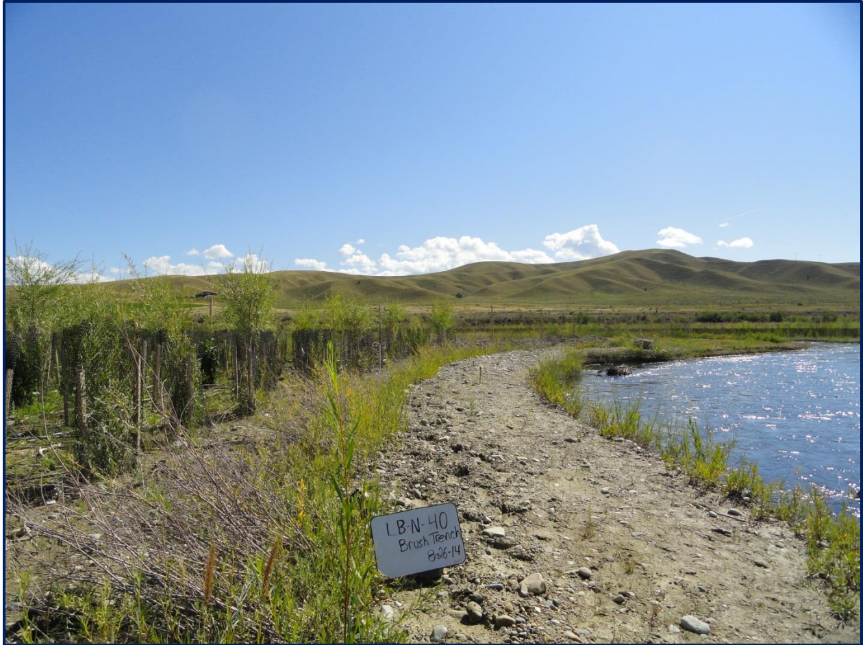
Figure 5-3. Brush trench streambank treatment in Phase 1 of the Clark Fork River Operable Unit.
