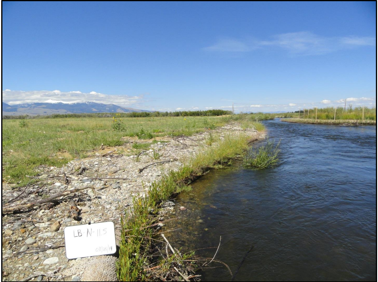
Figure 5-1. Single vegetated soil lift streambank treatment in Phase 1 of the Clark Fork River Operable Unit.
