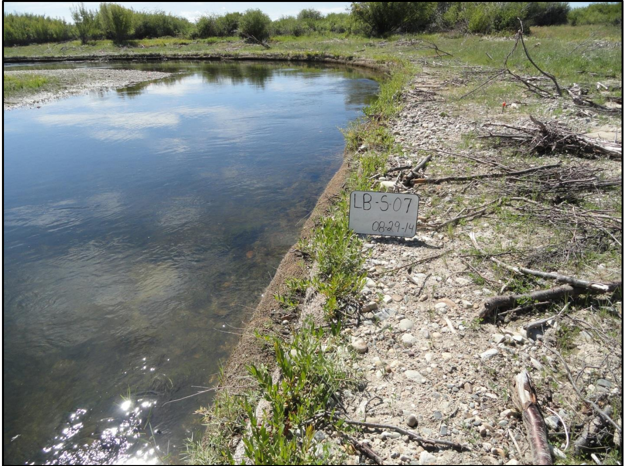
Figure 5-2. Double vegetated soil lift streambank treatment in Phase 1 of the Clark Fork River Operable Unit.
