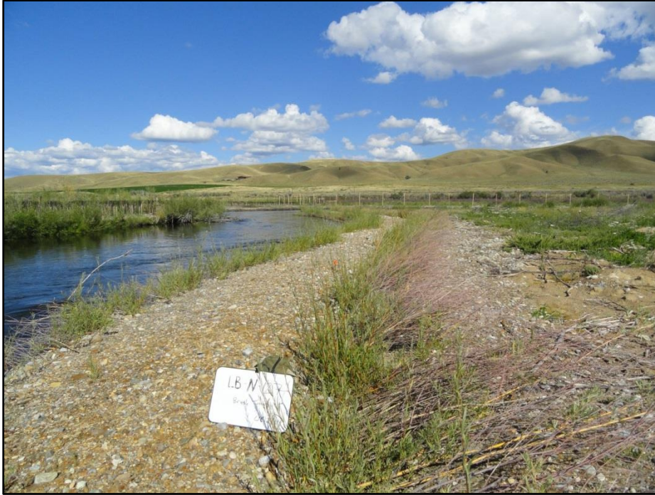
Figure 5-10. Example brush trench streambank treatment in Phase 1 of Reach A of the Clark Fork River Operable Unit, 2014.
