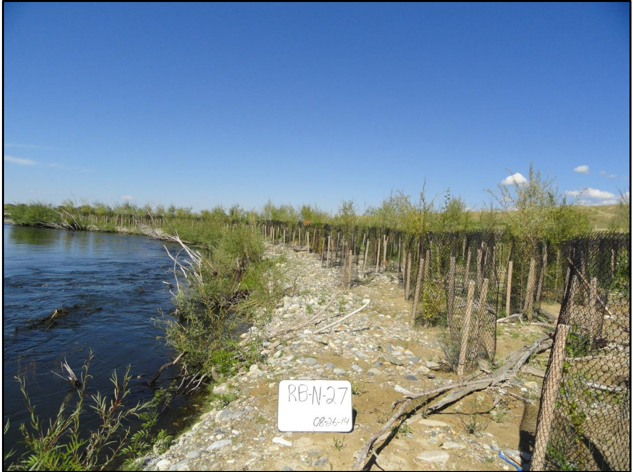
Figure 5-4. Preserve vegetation streambank treatment in Phase 1 of the Clark Fork River Operable Unit.
