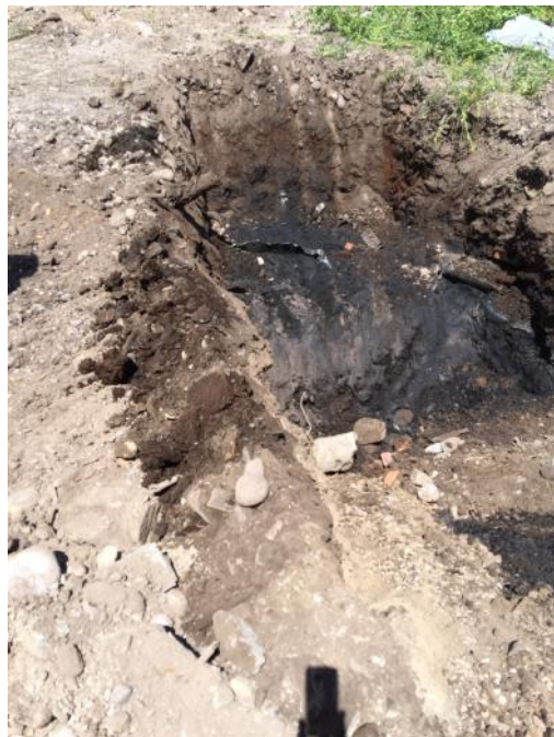
Photo 6. TP-4, first indication of buried tank
