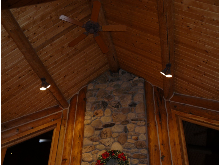
Junction of log wall at rock fireplace
