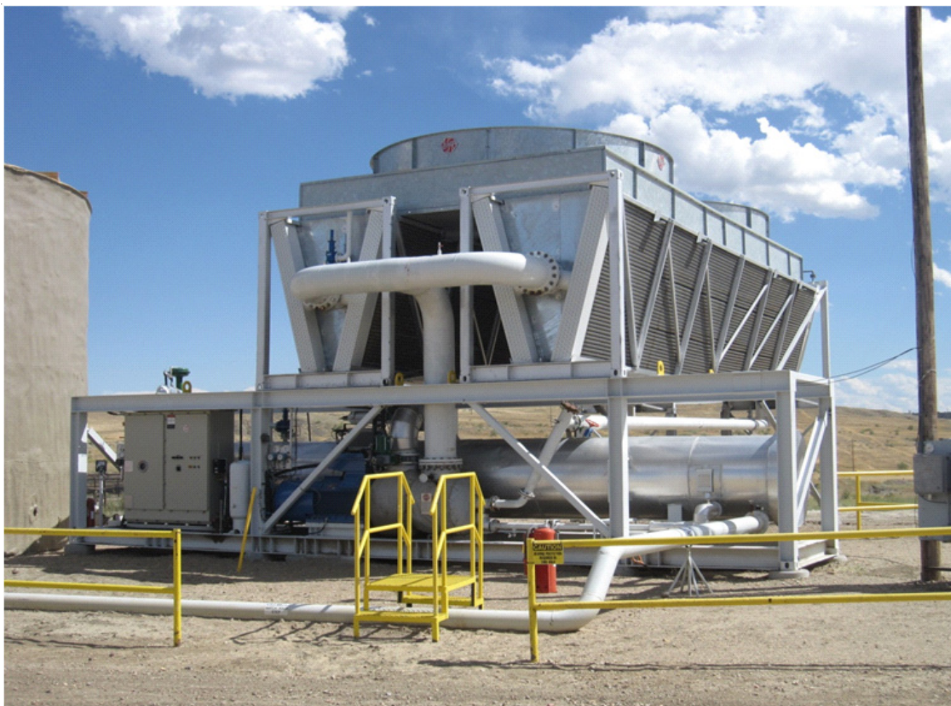
A binary generator at the Rocky Mountain Oilfield Testing facility near Casper, Wyoming. This power station uses 195 degree F water from an oil well to generate 250 kW of electricity.
