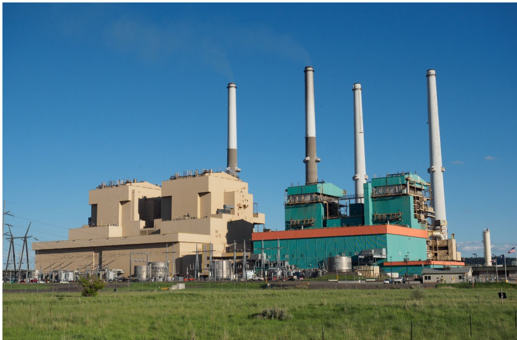
Figure 1.1. Colstrip Units 1–4 (from right to left).
