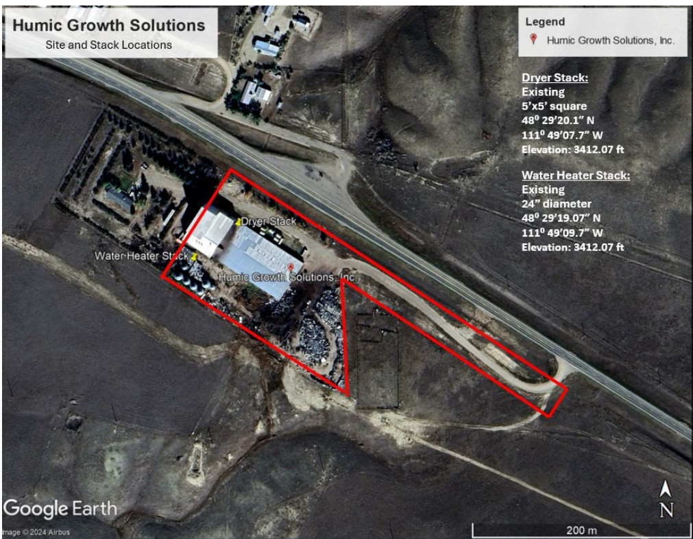
Figure 2. Detailed Aerial View
