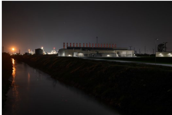
Figure 14-Entrance 02– All Lighting On
