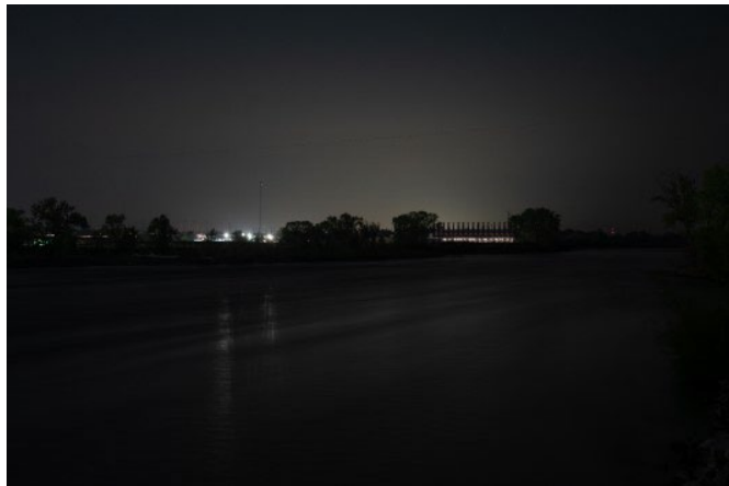
Figure 21- Bridge – Typical Nighttime Lighting
