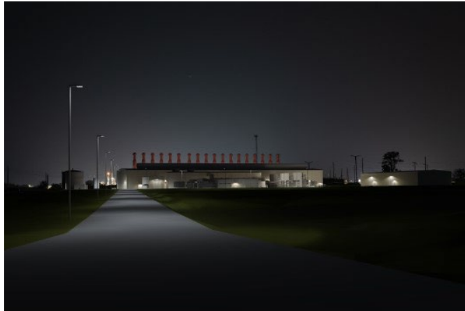
Figure 12- Entrance 01 – All Lighting On
