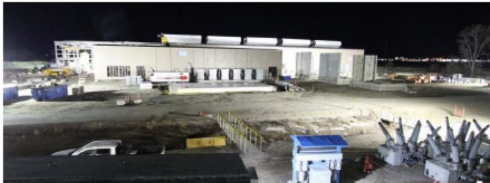
From construction trailers looking west
