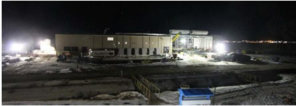
From construction trailers looking west
