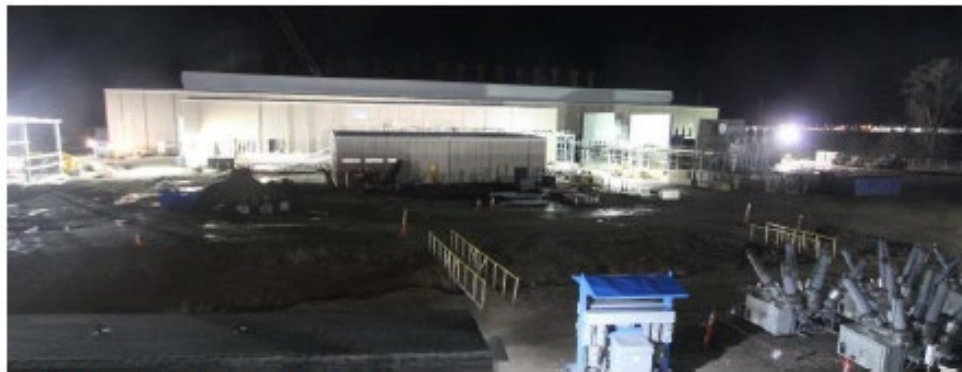
From construction trailers looking west
