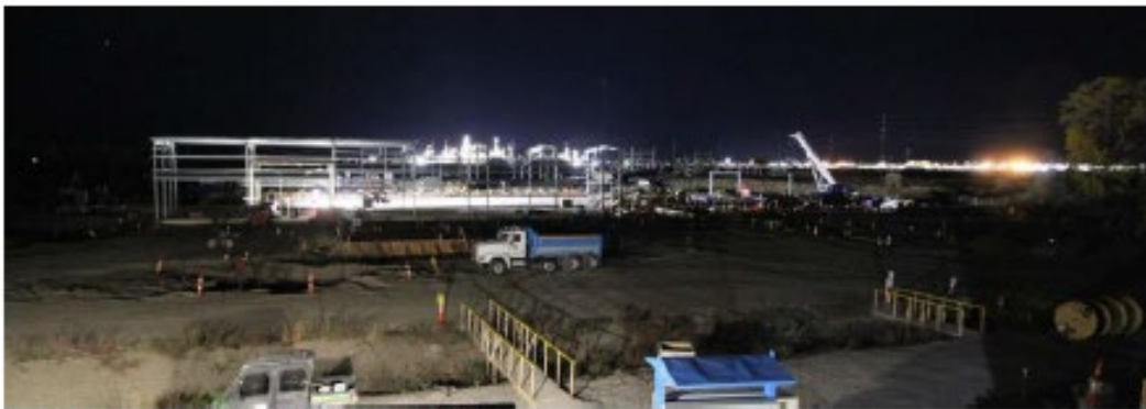
From construction trailers looking west
