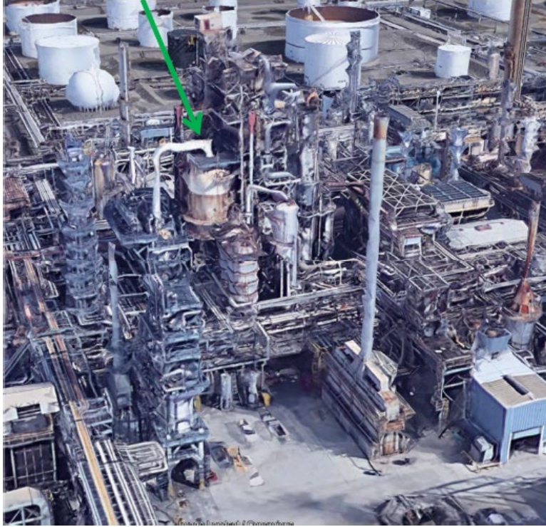
Figure 2: Phillips 66 Refinery, Green Arrow to FCCU
