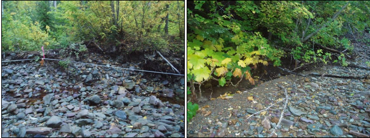
Figure B4-19. Typical eroding bank conditions in Marten Creek Reach 6-2.
