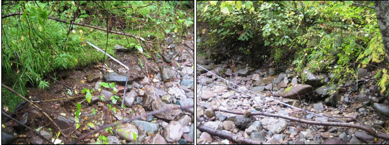
Figure B4-8. Typical eroding bank conditions in East Fork Elk Creek Reach 7-2.
