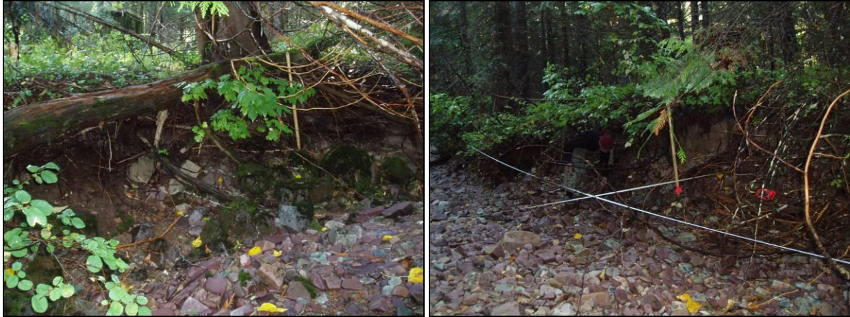
Figure B4-5. Typical eroding bank conditions in West Fork Elk Creek Reach 8-1.
