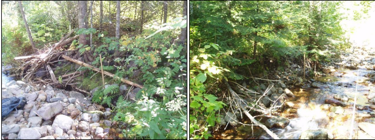
Figure B4-21. Typical eroding bank conditions in North Branch Marten Creek 8-1.
