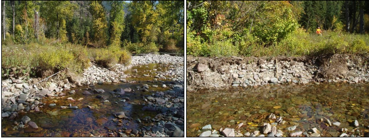
Figure B4-20. Typical eroding bank conditions in Marten Creek Reach 9-1.
