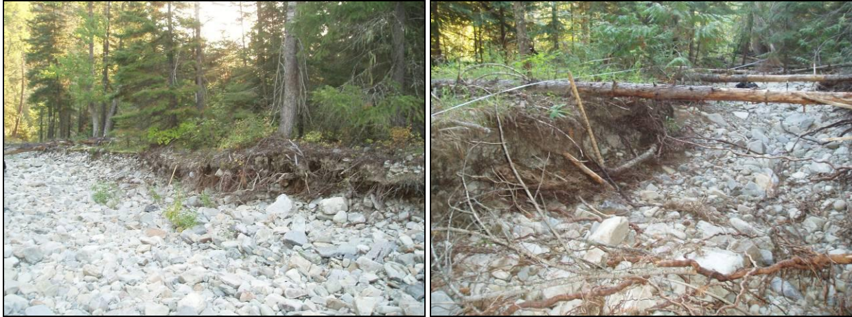
Figure B4-14. Typical eroding bank conditions in White Pine Creek Reach 8-3.
