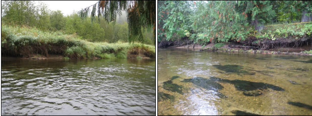
Figure B4-3. Typical eroding bank conditions in Bull River Reach 5-1.
