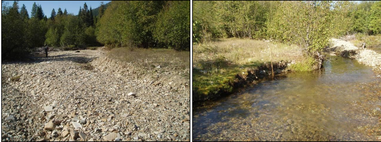
Figure B4-16. Typical eroding bank conditions in Swamp Creek Reach 20-1.
