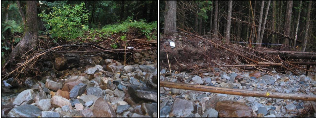
Figure B4-4. Typical eroding bank conditions in Dry Creek Reach 9-2.
