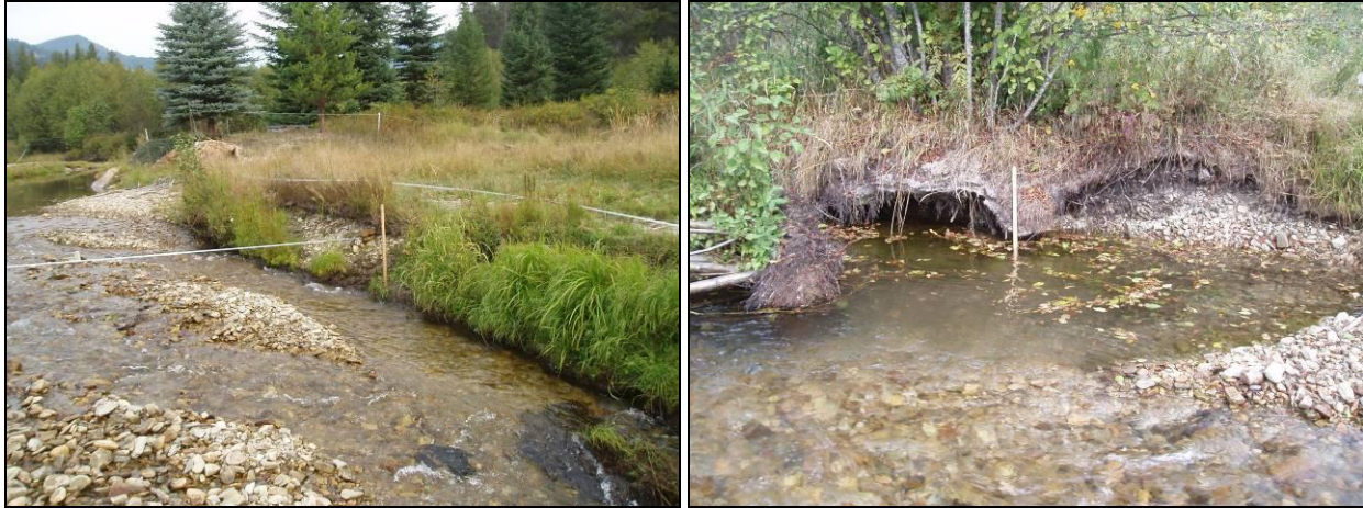
Figure B4-17. Typical eroding bank conditions in Swamp Creek Reach 21-1.
