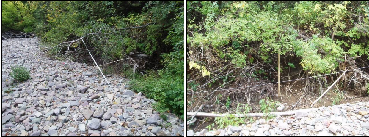
Figure B4-6. Typical eroding bank conditions in East Fork Elk Creek Reach 9-1.
