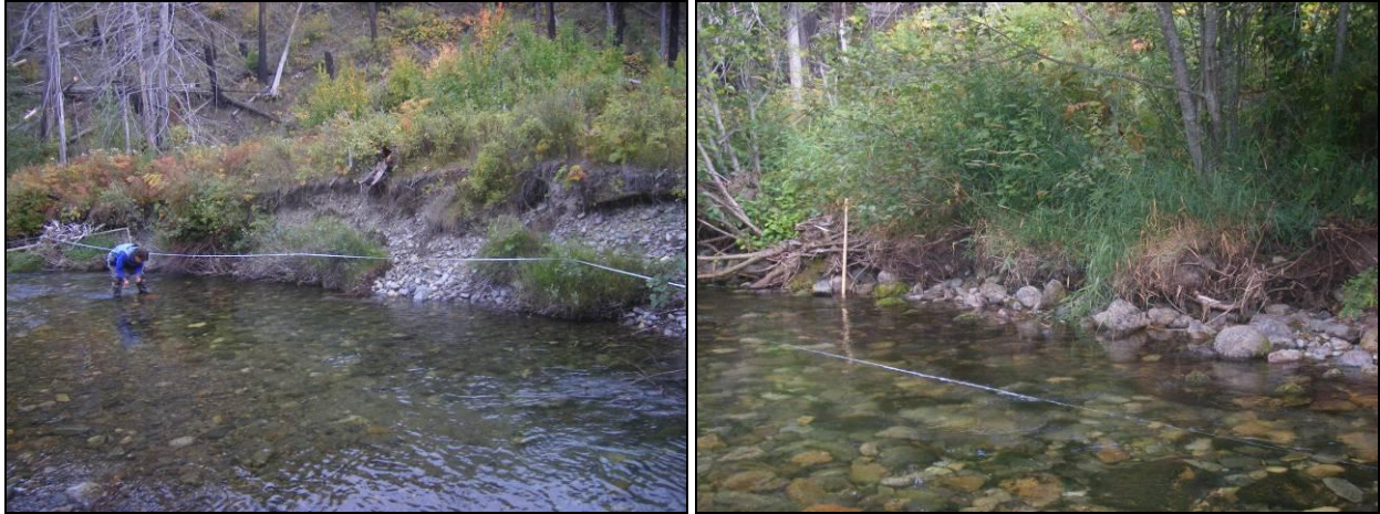
Figure B4-2. Typical eroding bank conditions in Bull River Reach 3-2.
