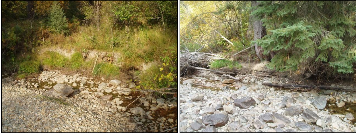
Figure B4-18. Typical eroding bank conditions in Swamp Creek Reach 22-3.
