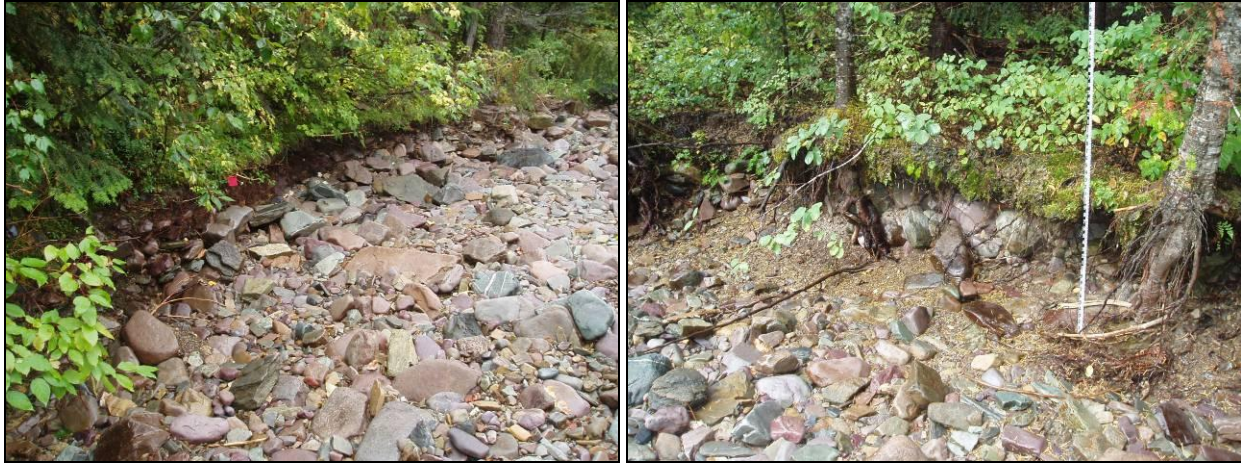
Figure B4-7. Typical eroding bank conditions in East Fork Elk Creek Reach 8-1.
