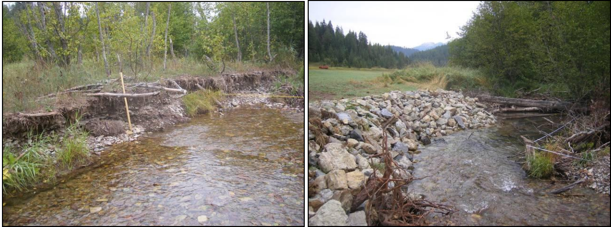
Figure B4-9. Typical eroding bank conditions in East Fork Elk Creek Reach 10-3.
