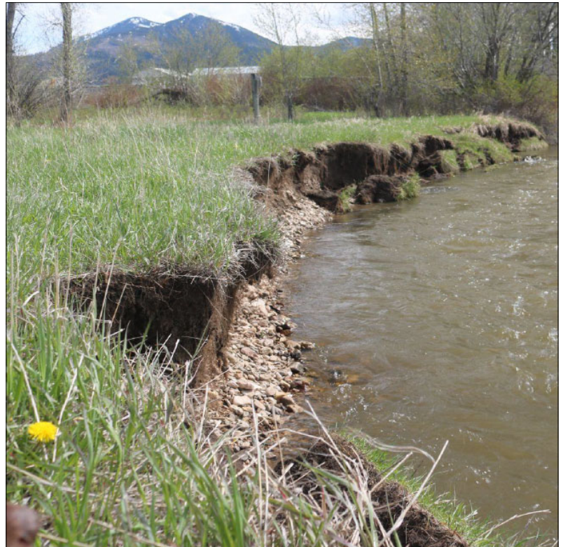
Eroding bank with shallow rooted vegetation at project site. (Photo: GWC)
