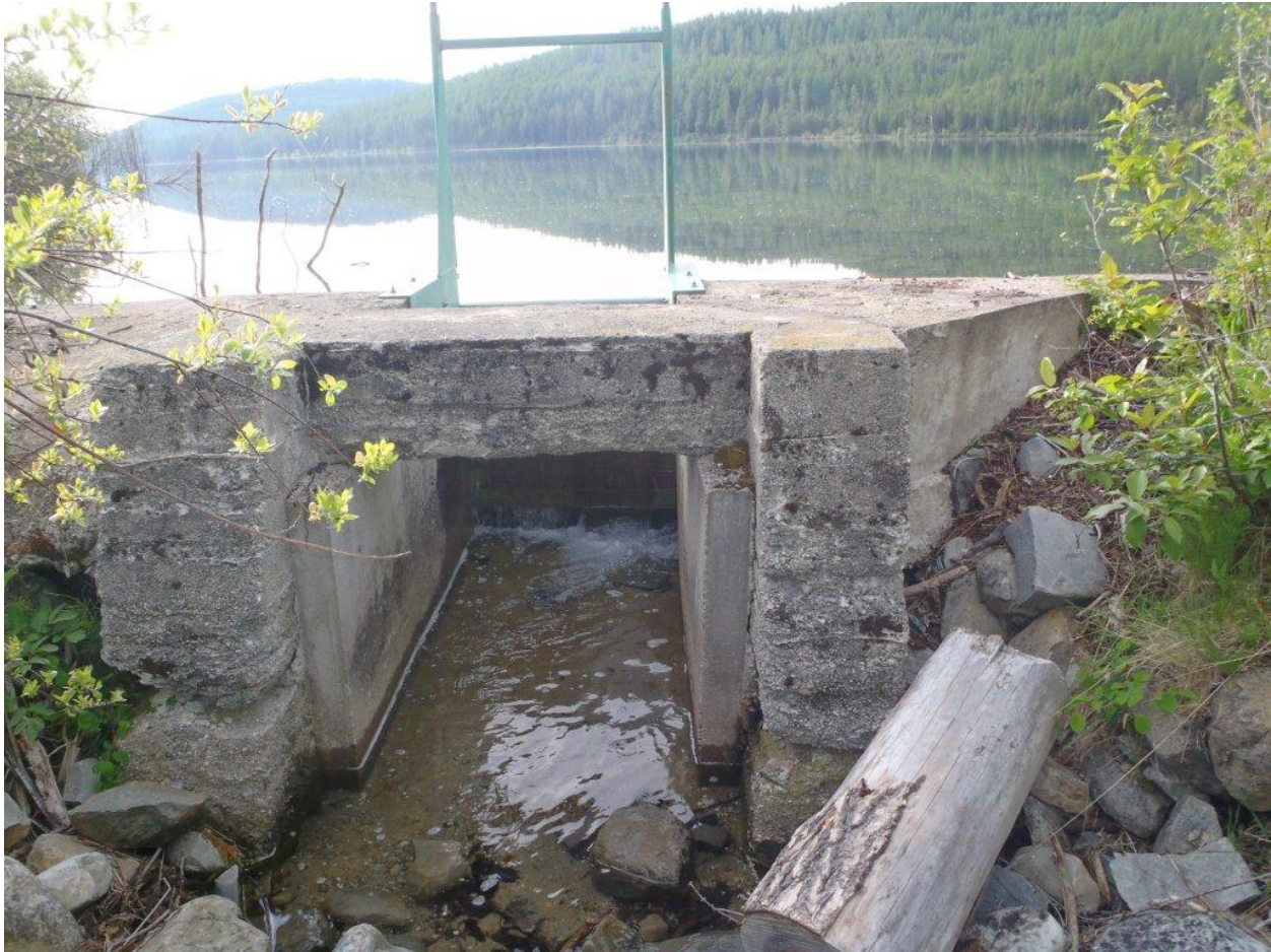
Figure 2. The outlet of McGregor Lake at Palm Dam.
