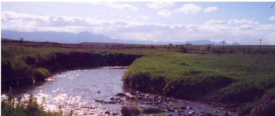
Figure 3-9. Riparian removal and apparent downcutting on Willow Creek.
