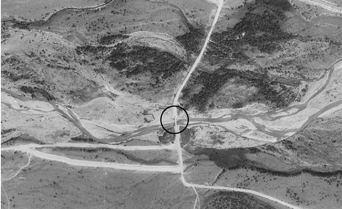
Figure 4-13. An undersized highway structure (bridge in circle) on the upper Teton River that limits floodway access and creates a constricted stream channel (photo scale is 1:5,000).
