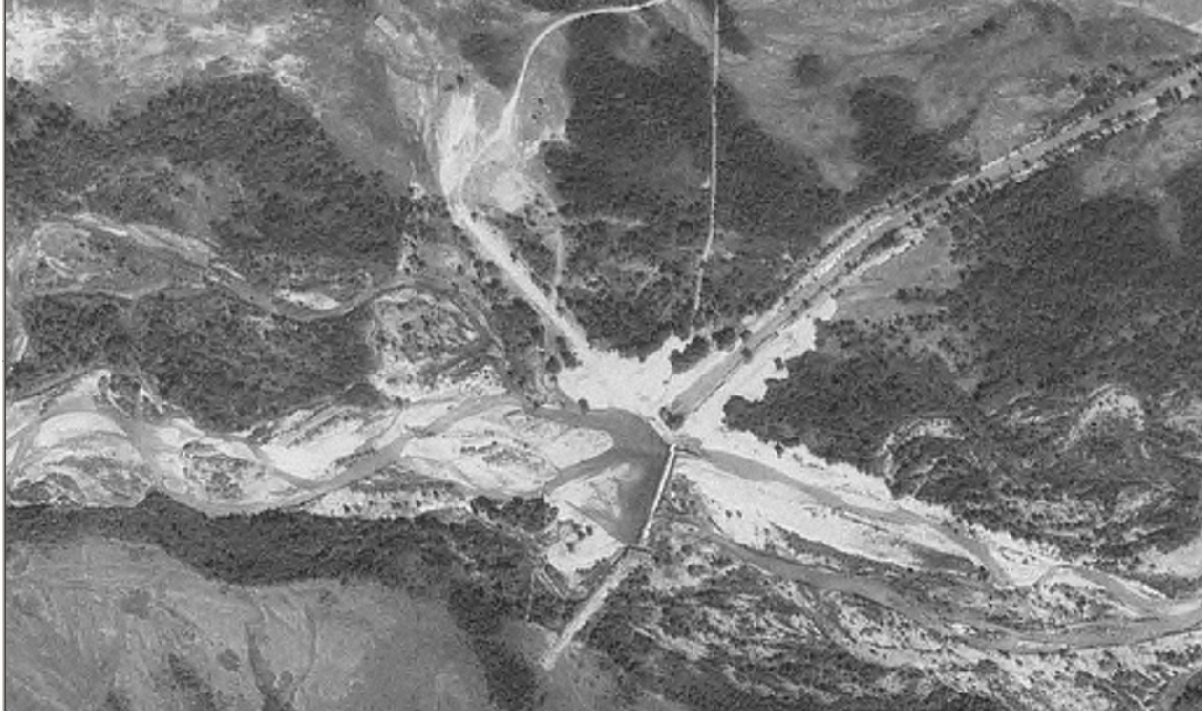
Figure 4-12. Example of an instream diversion structure on the upper Teton River (photo scale is 1:4,000).
