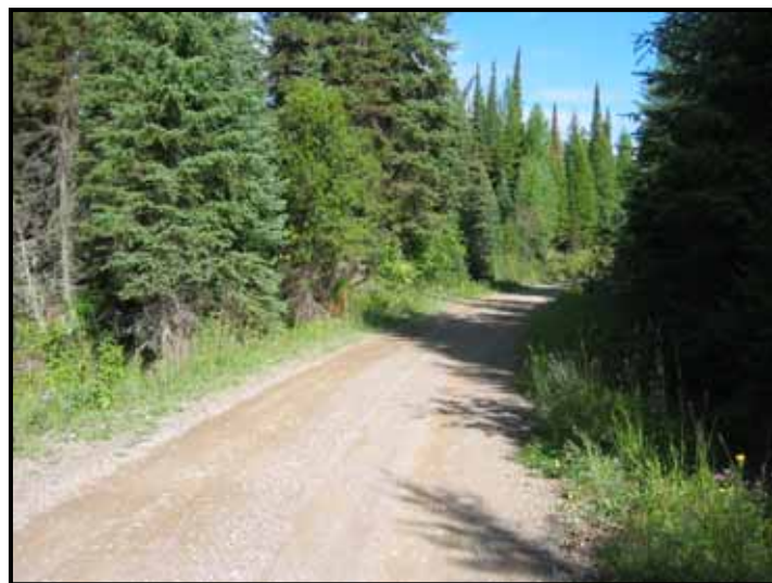
Photo 5-2. Example of a road considered to have a high potential for erosion and sediment delivery.
