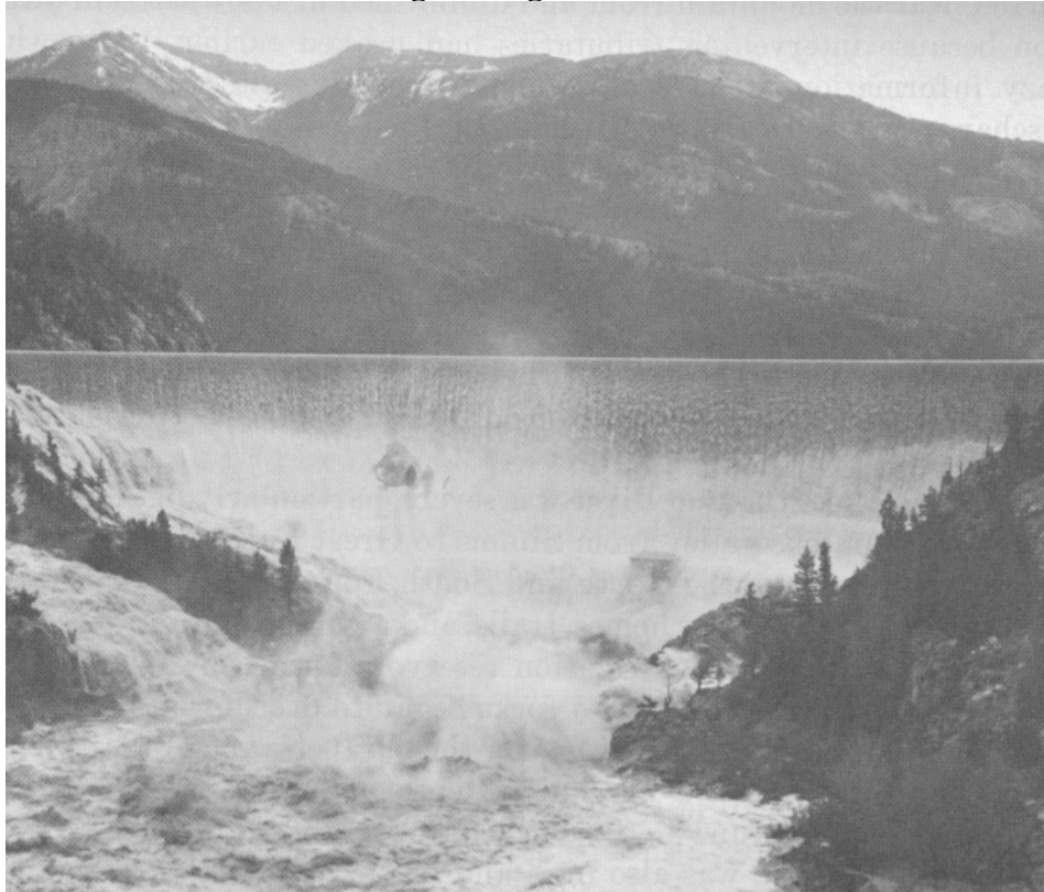
Figure 9-18. Gibson Dam over Flowing During 1964 Flood.
