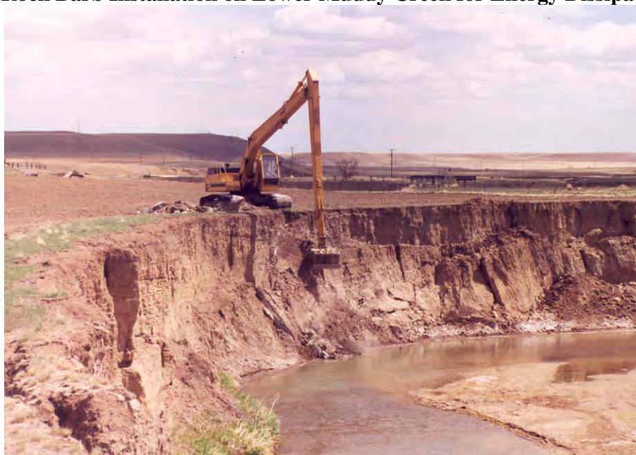
Figure 9-8. Rock Barb Installation on Lower Muddy Creek for Energy Dissipation (1996).
