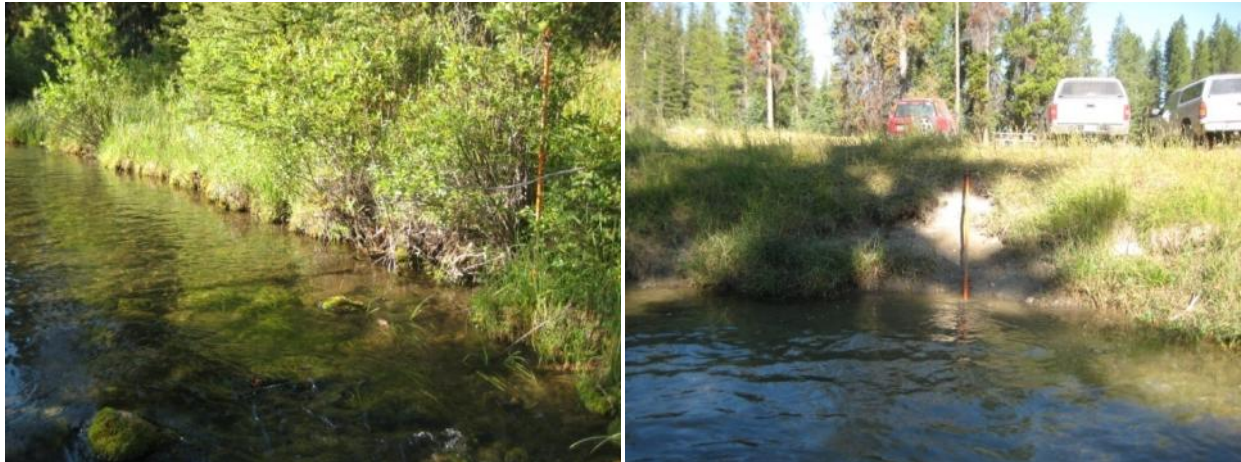
Figure C4-5. Typical eroding streambank conditions in East Fork Rock Creek Reach 01-02.
