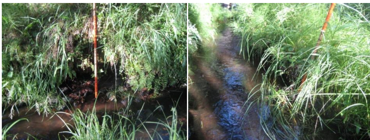
Figure C4-12. Typical eroding streambank conditions in Scotchman Gulch Reach 08-01.
