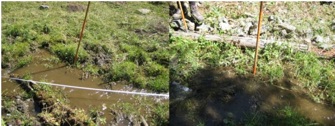
Figure C4-14. Typical eroding streambank conditions in South Fork Antelope Creek 06-01.
