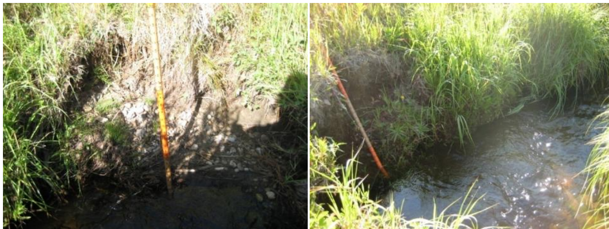
Figure C4-10. Typical eroding streambank conditions in Miners Gulch Reach 14-02.
