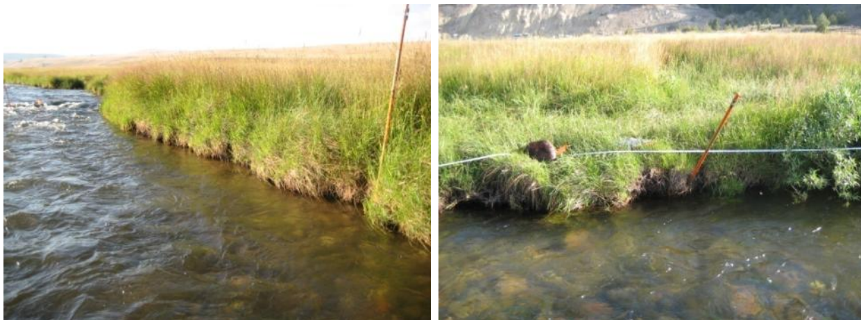
Figure C4-6. Typical eroding streambank conditions in East Fork Rock Creek Reach 03-03.
