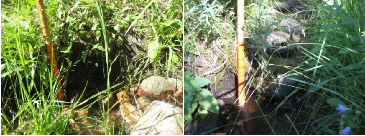
Figure C4-8. Typical eroding streambank conditions in Flat Gulch Reach 13-01.
