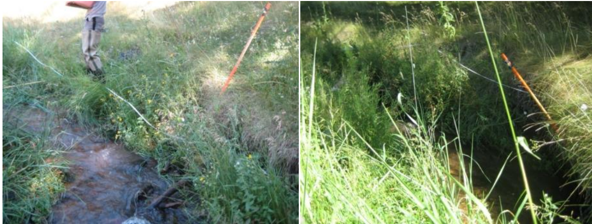
Figure C4-16. Typical eroding streambank conditions in Sluice Gulch Reach 14-01.
