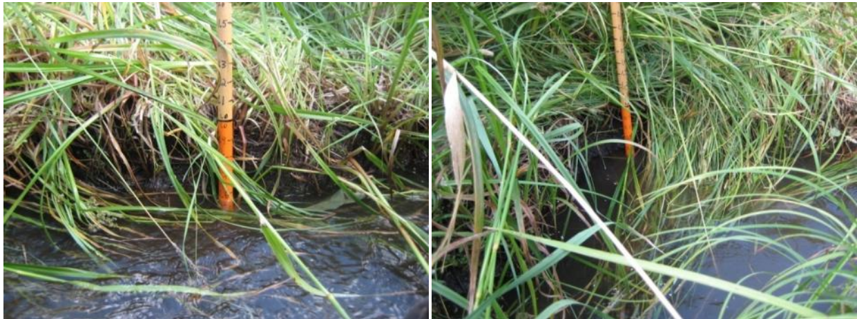
Figure C4-13. Typical eroding streambank conditions in Scotchman Gulch Reach 16-01.
