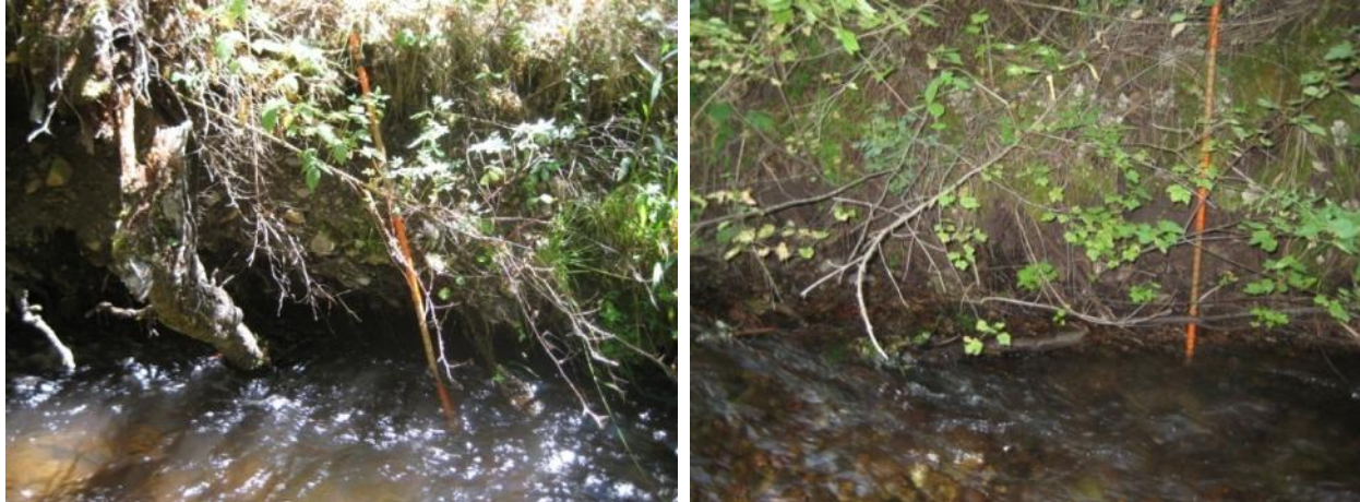
Figure C4-3. Typical eroding streambank conditions in Brewster Creek Reach 05-01.
