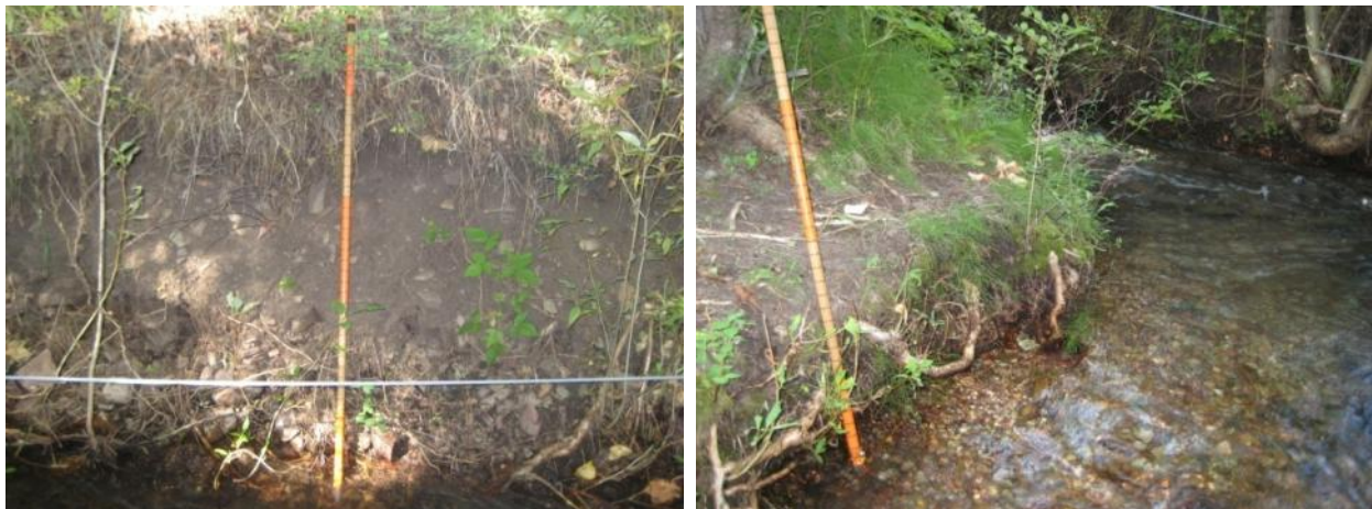
Figure C4-4. Typical eroding streambank conditions in Brewster Creek Reach 06-01.
