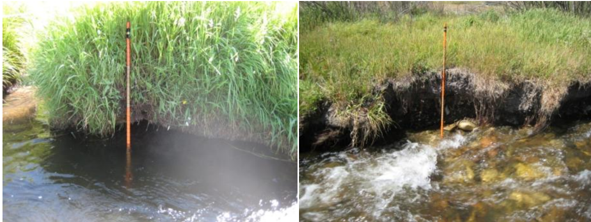
Figure C4-18. Typical eroding streambank conditions in Upper Willow Creek Reach 11-05.
