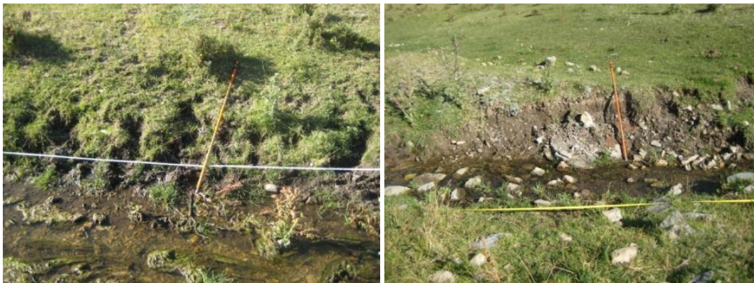
Figure C4-1. Typical eroding streambank conditions in Antelope Creek Reach 07-01.
