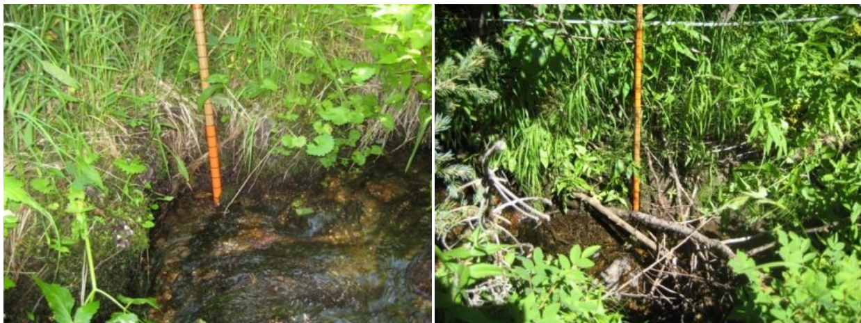
Figure C4-9. Typical eroding streambank conditions in Miners Gulch Reach 10-02.
