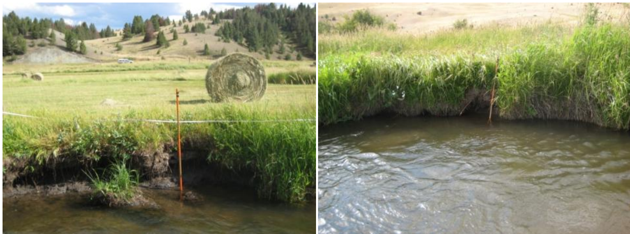
Figure C4-19. Typical eroding streambank conditions in Upper Willow Creek Reach 15-01.
