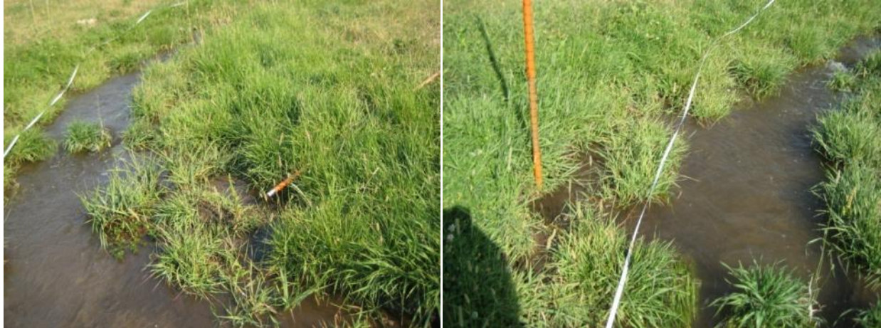
Figure C4-2. Typical eroding streambank conditions in Antelope Creek Reach 21-01.
