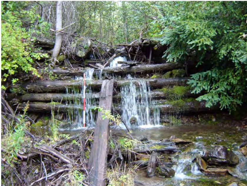
Photo 4-6. Fish Passage Barrier in Little McCormick Creek.
