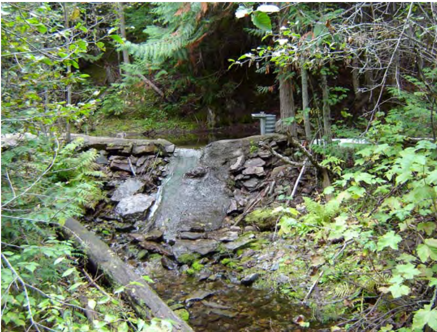
Photo 4-10. Fish Passage Barrier on Kennedy Creek.
