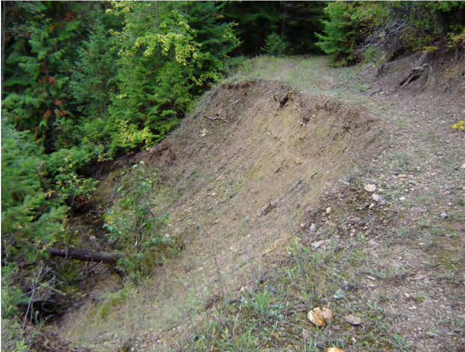
Photo 4-9. Road Failure on Kennedy Creek.
