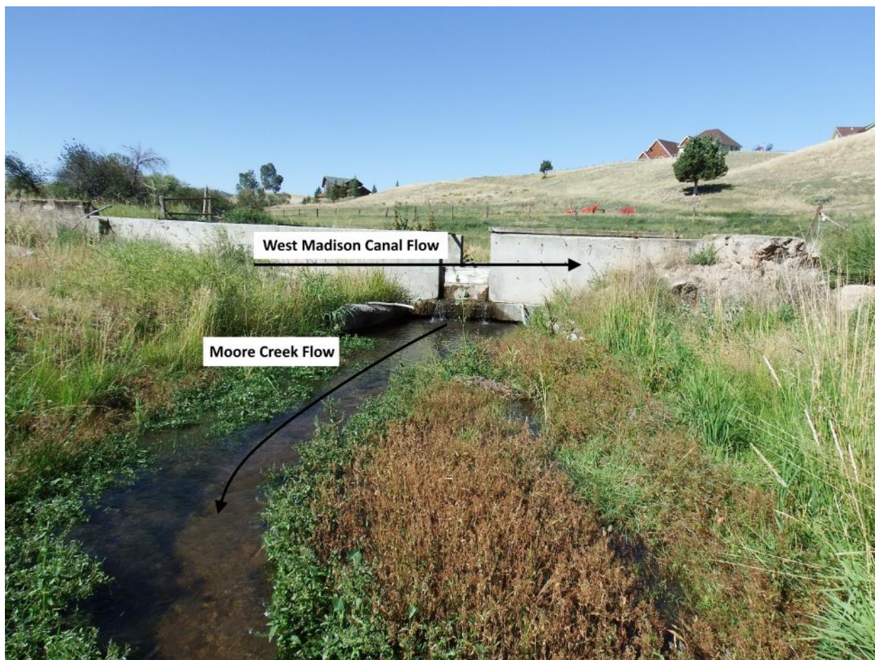
Figure 6-22. Photo showing West Madison Canal crossing Moore Creek and mixing through leaky check-boards in the center of the photo. Headgate releases water into Moore Creek to the left of photo (off photo).
