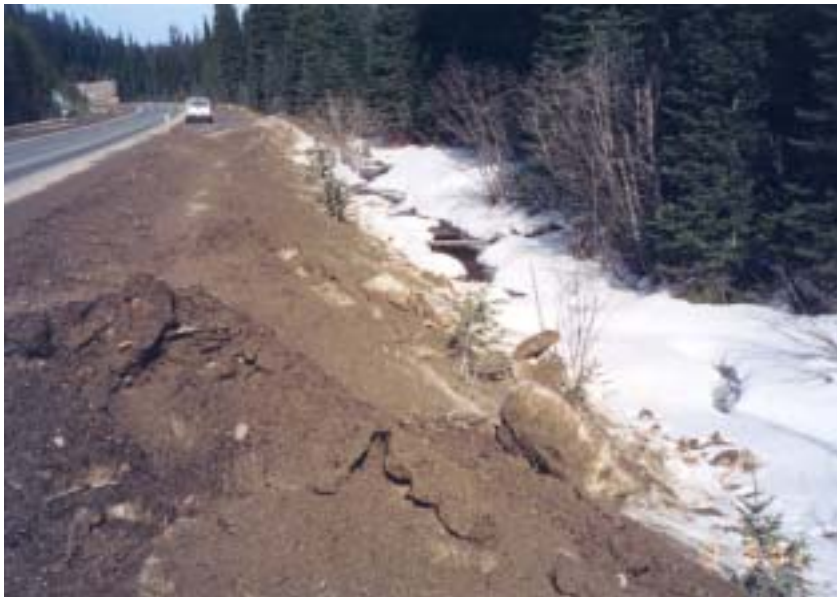
Figure 10. U.S. Highway 12 along W.F. Lolo Creek.
