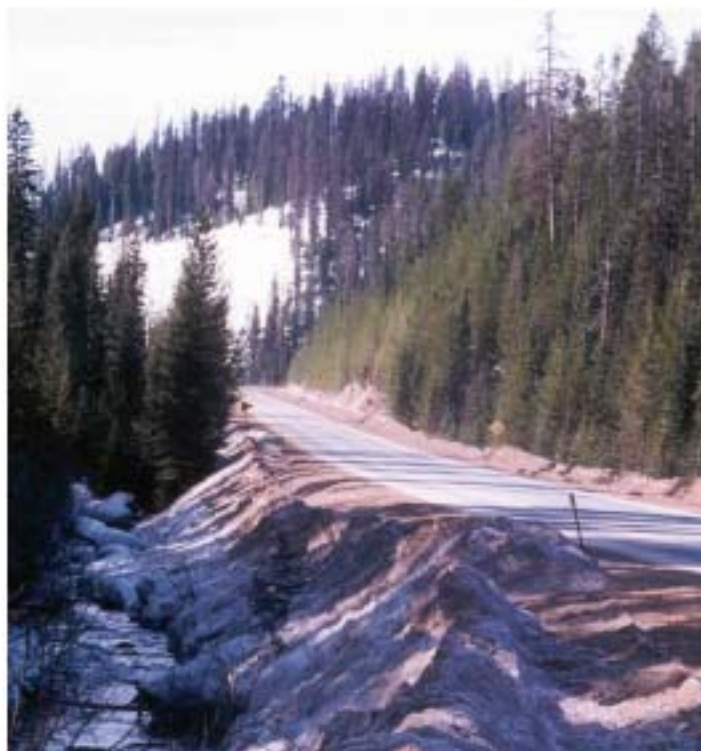
Figure 11. U.S. Highway 12 along W.F. Lolo Creek.
