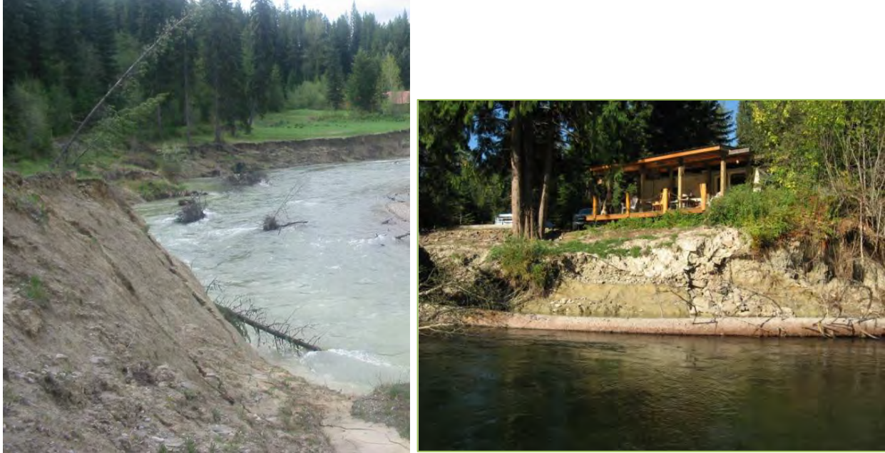
Figure 5-3. Actively eroding streambanks on Lake Creek that have worsened by removal of riparian vegetation and development. Left photo courtesy of K. Newgard, Kootenai National Forest, 2009.
