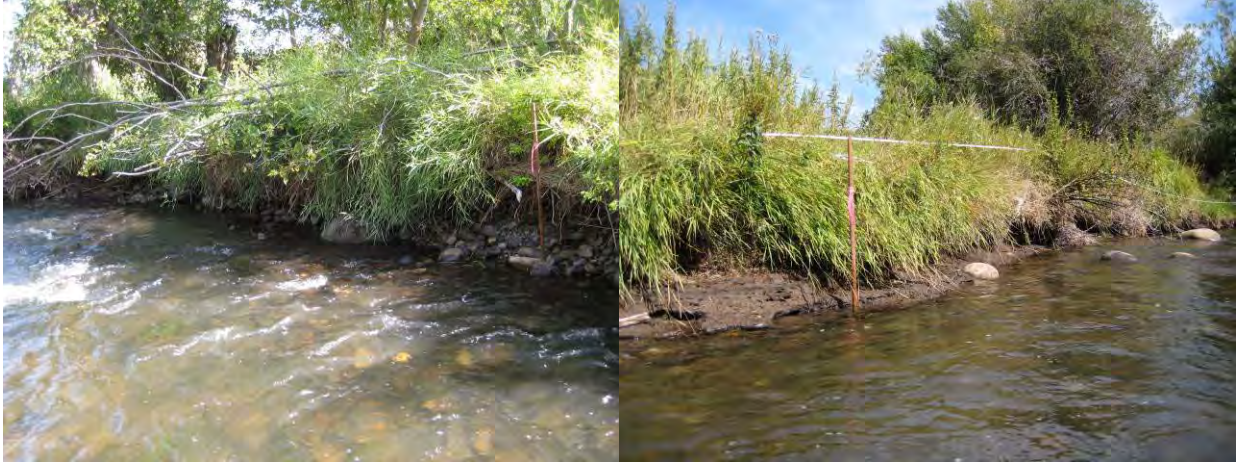
Figure 4-15. Typical eroding streambank conditions in Flint Creek Reach 18-05.
