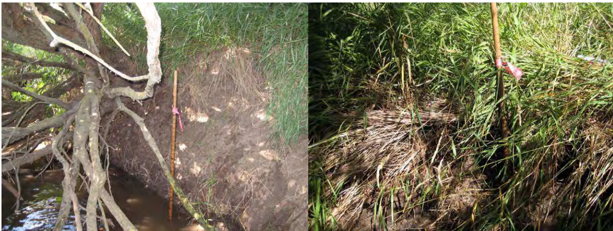
Figure 4-3. Typical eroding streambank conditions in Barnes Creek Reach 13-03.
