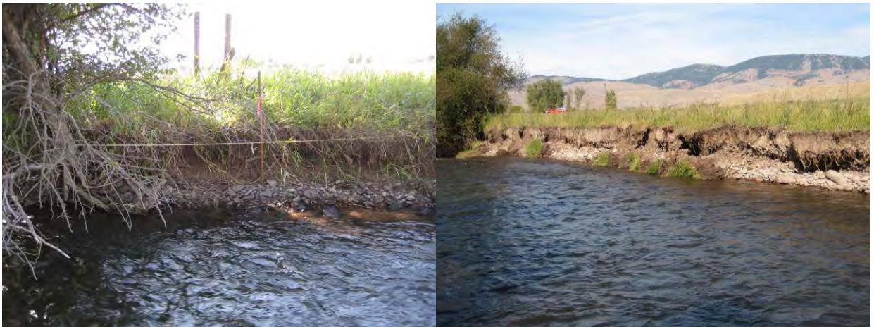
Figure 4-16. Typical eroding streambank conditions in Flint Creek Reach 19-01.
