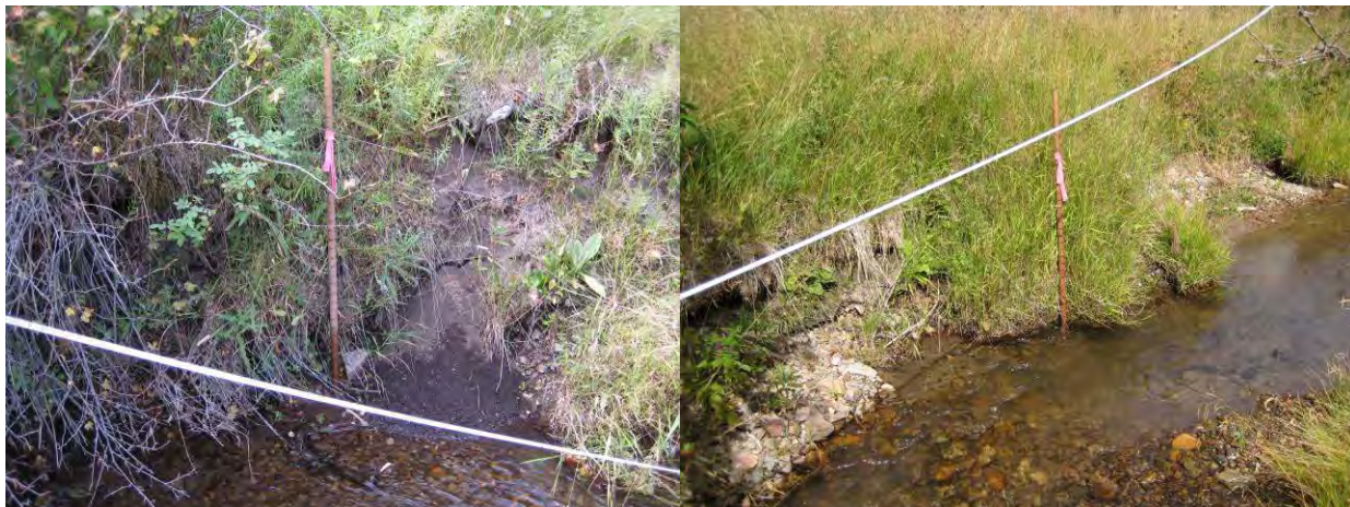
Figure 4-21. Typical eroding streambank conditions in Smart Creek Reach 18-01-2.
