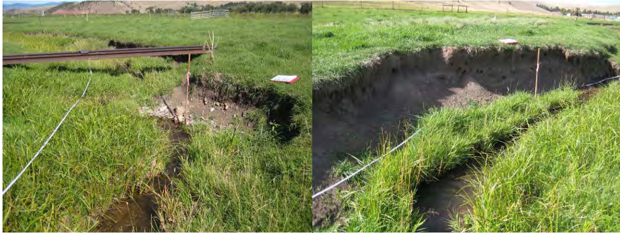
Figure 4-22. Typical eroding streambank conditions in Smart Creek Reach 21-01.
