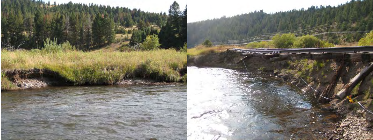
Figure 4-11. Typical eroding streambank conditions in Flint Creek Reach 11-01.
