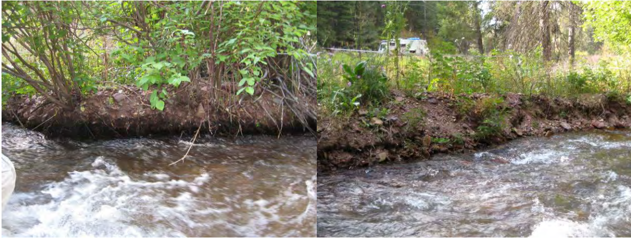
Figure 4-9. Typical eroding streambank conditions in Flint Creek Reach 06-02.
