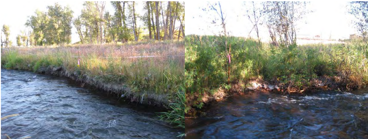
Figure 4-10. Typical eroding streambank conditions in Flint Creek Reach 09-02.
