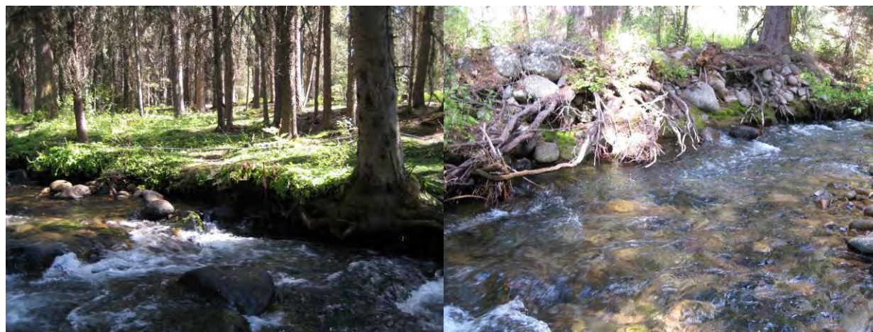
Figure 4-4. Typical eroding streambank conditions in Boulder Creek Reach 16-01.
