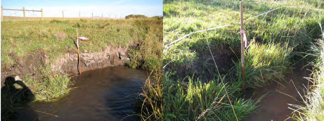
Figure 4-2. Typical eroding streambank conditions in Barnes Creek Reach 13-01.
