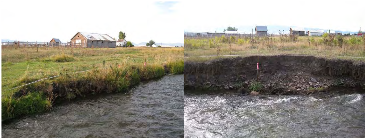
Figure 4-18. Typical eroding streambank conditions in Lower Willow Creek Reach 02-05.
