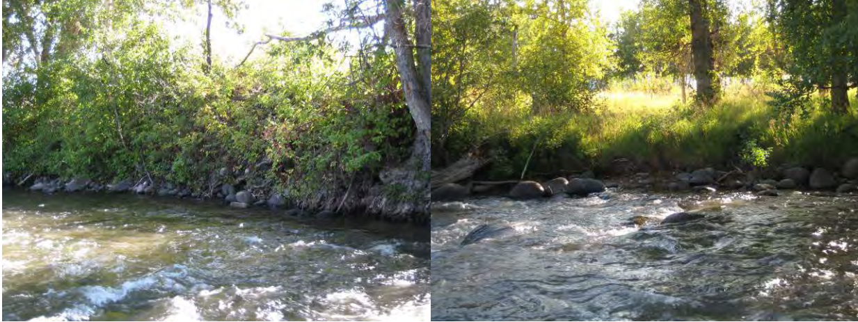
Figure 4-13. Typical eroding streambank conditions in Flint Creek Reach 17-01.
