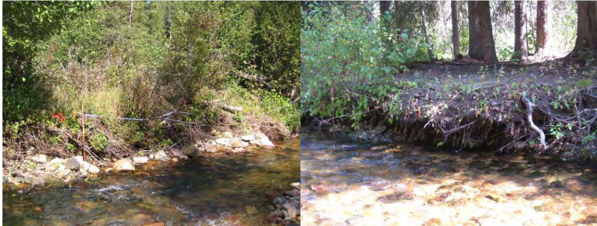
Figure 4-5. Typical eroding streambank conditions in Boulder Creek Reach 21-02.
