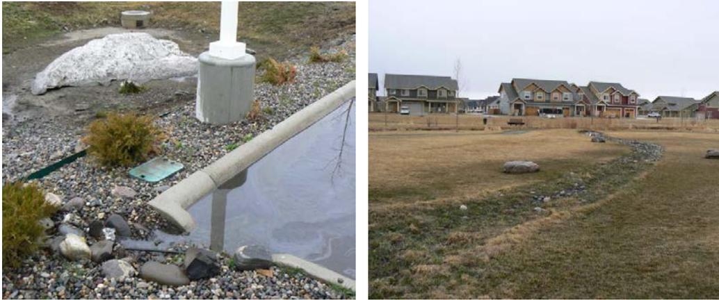
**Figure 9-1. Stormwater BMPs: Parking lot designed to drain into a swale and a mixed use development**
