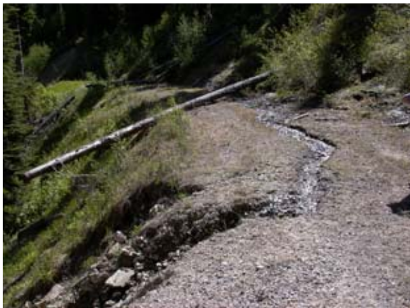
Figure 4-4. Active stream eroding road prism on Road 5278.
