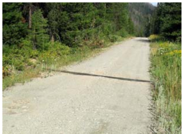
Figure 4-6. Example of BMP to divert water from the road surface.
