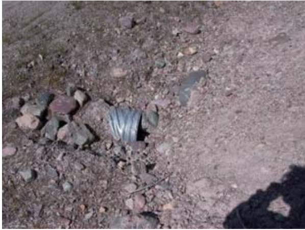
Figure 4-3. Plugged culvert at Road 1693.
