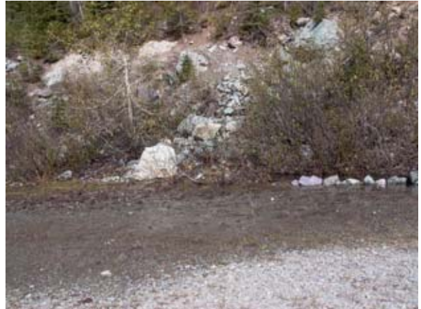
Figure 4-5. Plugged culvert on Road 1604.
