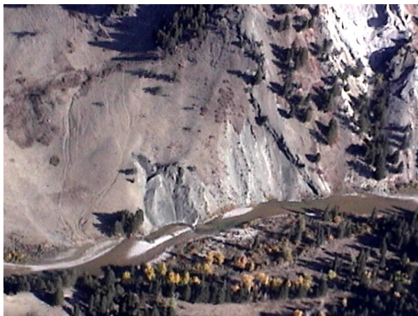
Figure 3-31. Slumps in Dearborn Mainstem Reach 6
