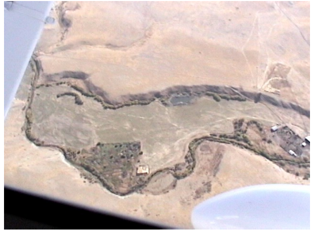
Figure 3-10. Central Portion of South Fork SF1 ‘Poor’
