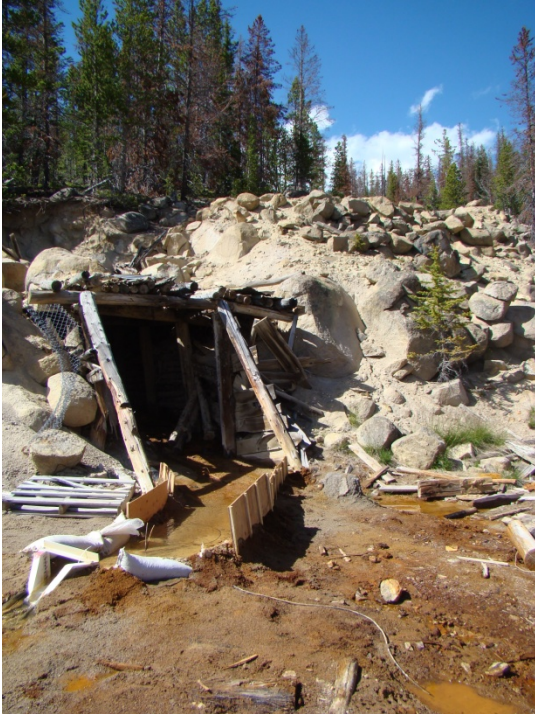
Figure 5-1. The iron oxide precipitation effects of ARD at the lower Crystal Mine adit discharge
