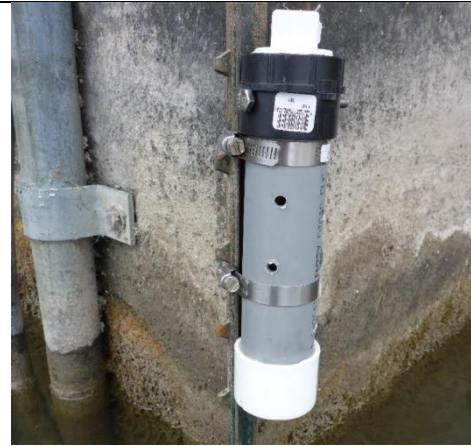
Figure 26. Fencepost deployment at bridge abutment closeup
