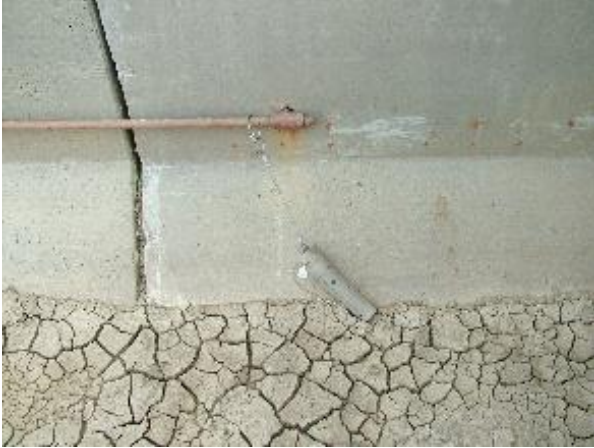
Figure 23. Culvert At a site known to go dry.
