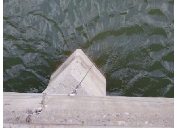
Figure 24. Cable attachment to a bridge using stainless steel cable, ferrules, thimble, threaded clevis hardware.
