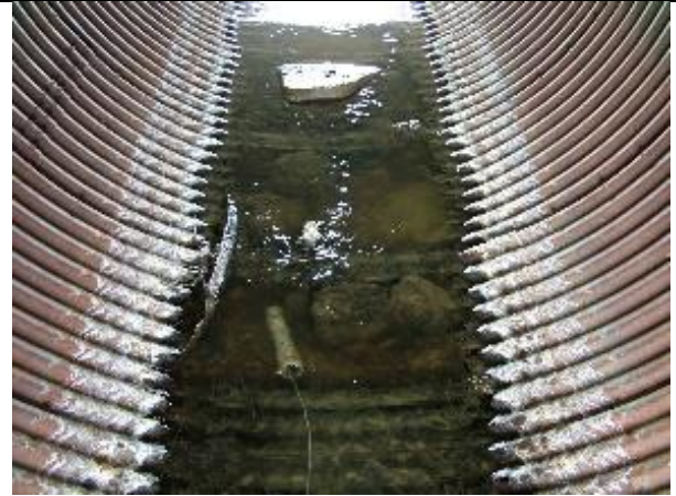
Figure 20. Culvert deployment designed to only capture flowing water data.
