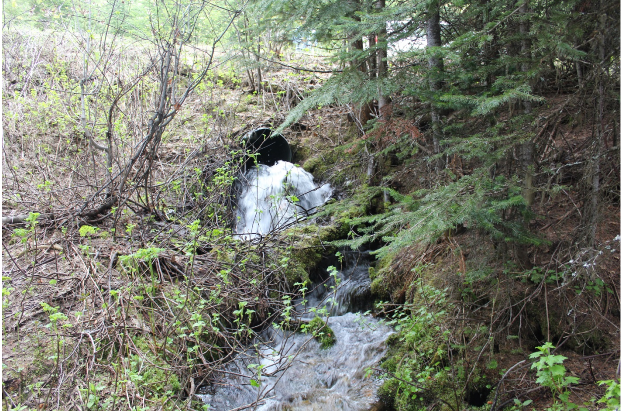
Figure 4 Miller Creek Headwaters: Though the headwaters are relatively healthy, undersized culverts carry high velocity flows that serve as a barrier to fish migration
