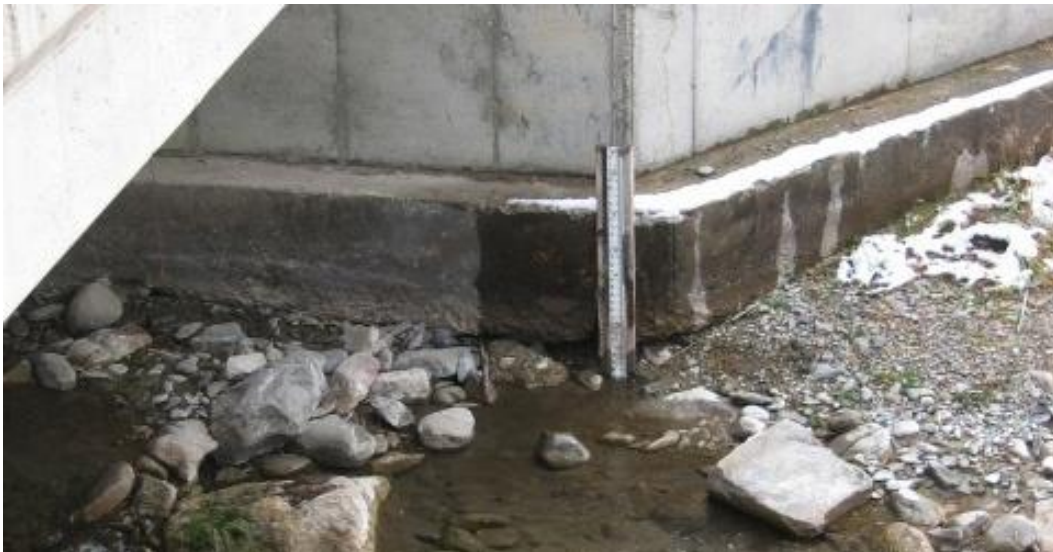
Figure 19. Exposed bridge pier footer indicating channel bed degradation, Reach 10. (P. Skidmore photo, 2012)
