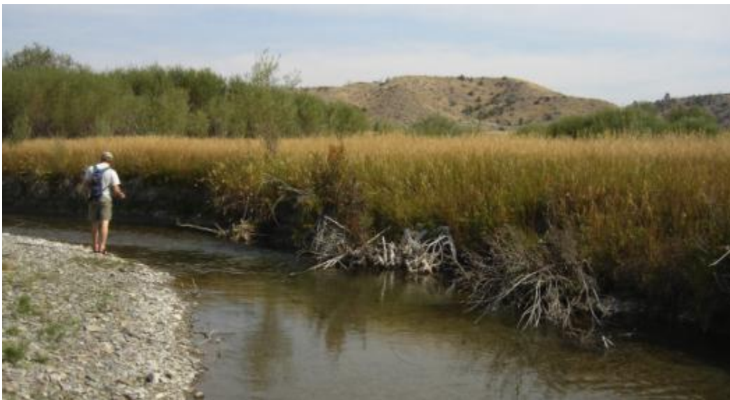
Figure 13. Juniper revetments have partially washed away, though they still provide some protection at the toe of the bank, Reach 13. (R. Spoon photo, 2012)
