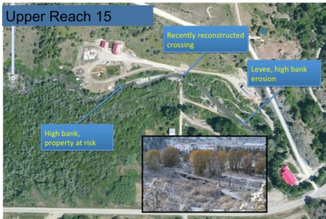
Figure 23. Example of concentrated infrastructure within an unstable stream reach immediately below the Deep Creek canyon in Reach 15.
