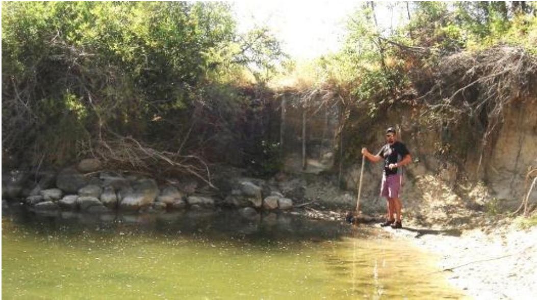
Figure 19. Exposed bridge pier footer indicating channel bed degradation, Reach 10. (P. Skidmore photo, 2012)
