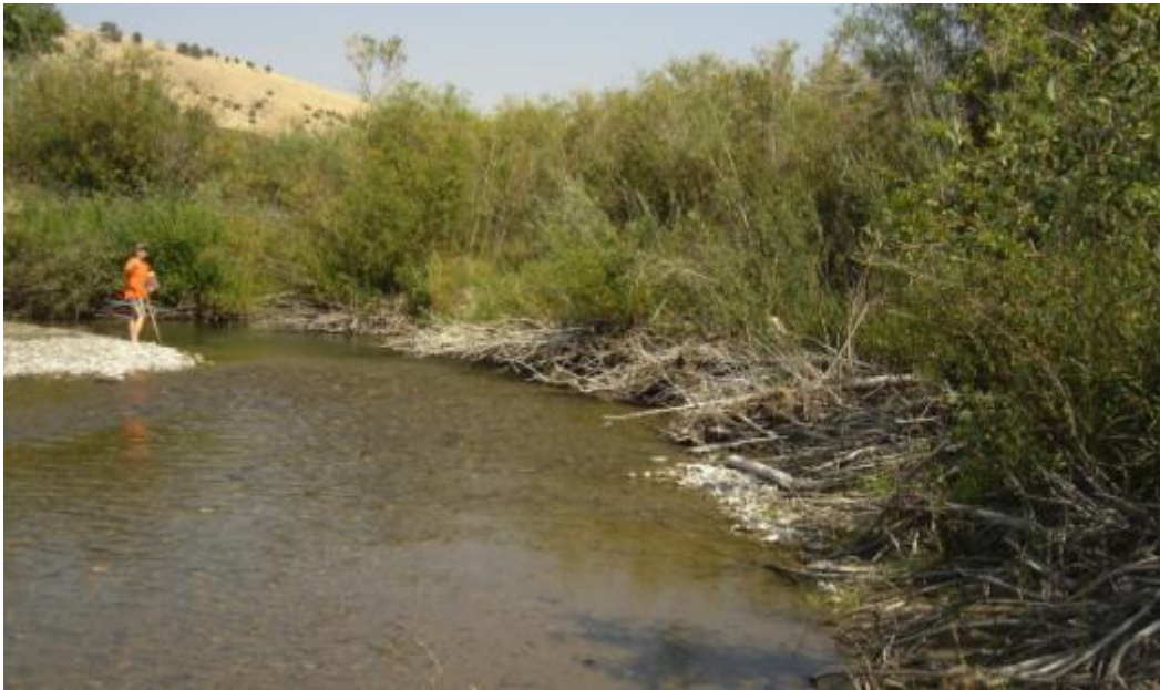
Figure 12. Juniper revetment with effective revegetation, Reach 11. (R. Spoon photo, 2012)
