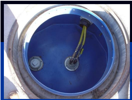
Figure 2: Typical supply and return line for an emergency generator or heating oil tank system
