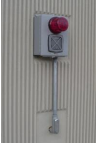
Figure 1. High Level Alarm
