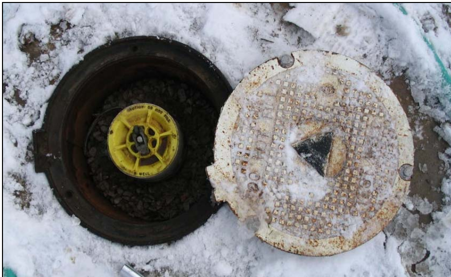
Monitoring Well Cap and Cover
