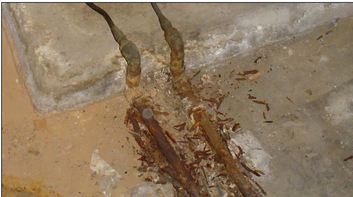
Corroded Metal Piping
