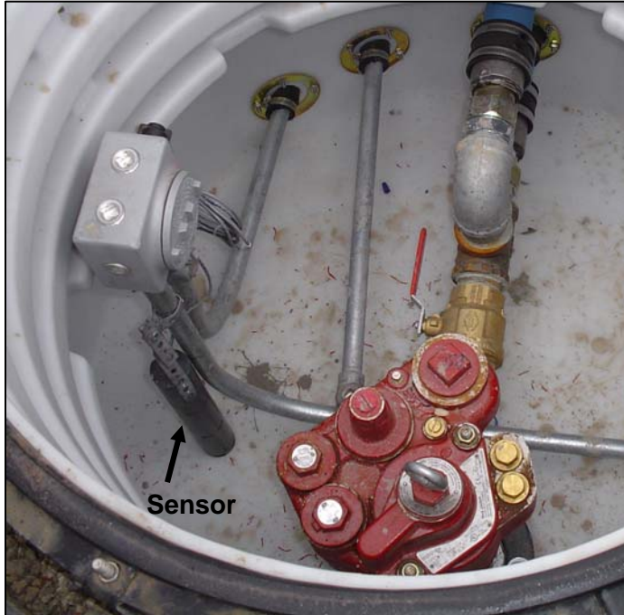
Sample Sump of Continuous Interstitial Monitoring
