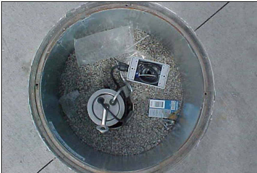
Interstitial Monitor Probe for a Double Walled Tank. (Notice the wires for reporting back to the ATG)
