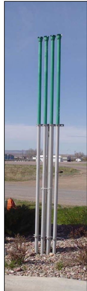
Vent Stacks with rain caps on top
