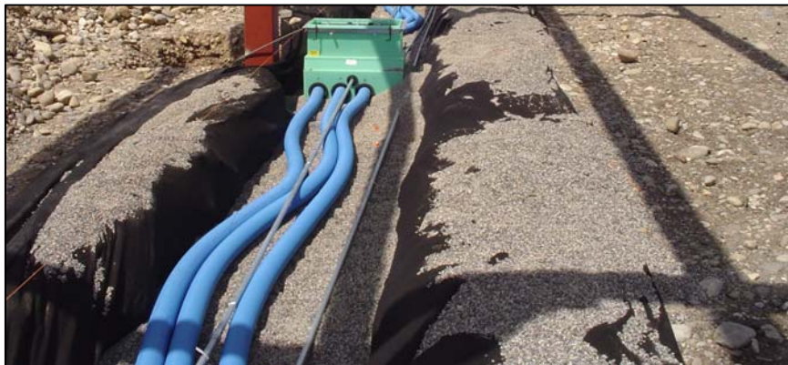
UST Piping with Interstitial Monitoring as Leak Detection
