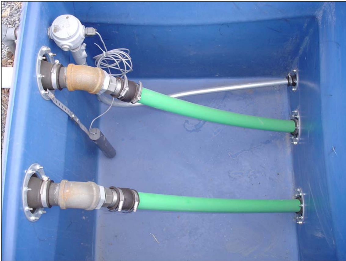
Transition Sump for Aboveground Piping to Underground Piping
