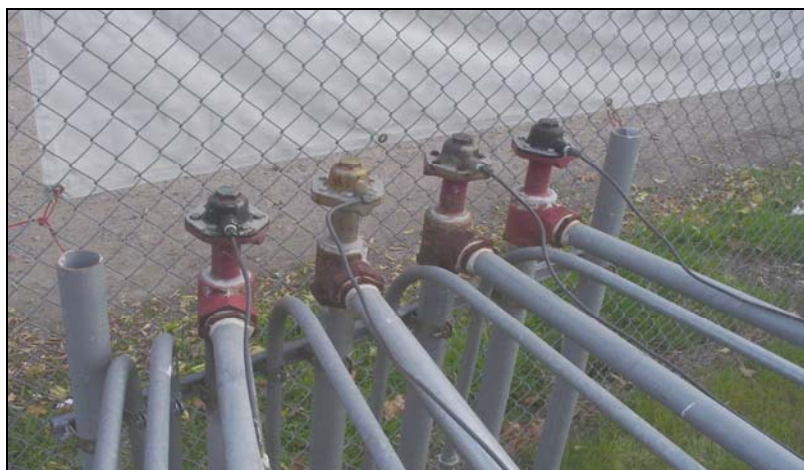
Mechanical LLD's set up for underground piping from an aboveground storage tank.
