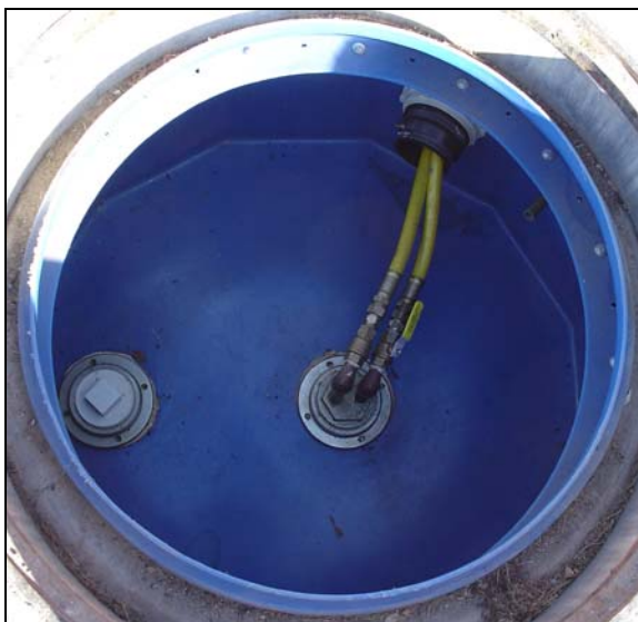
Containment Sump of a Suction system (U.S. Suction)
