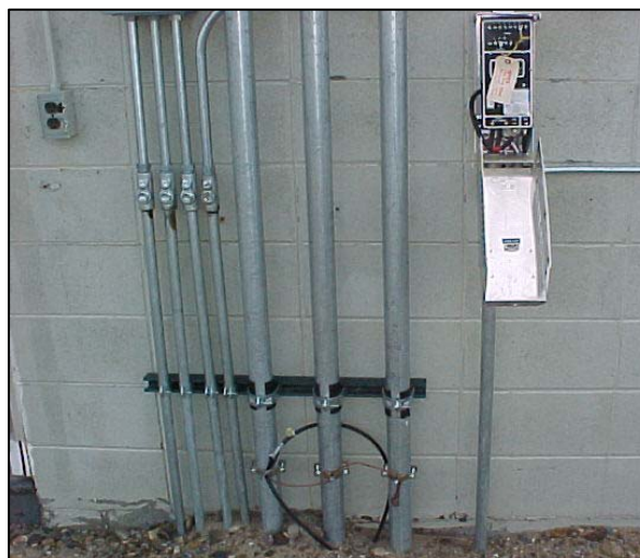
Rectifier Box and Impressed current on vent stacks
