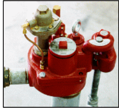
Mechanical LLD installed on a STP
