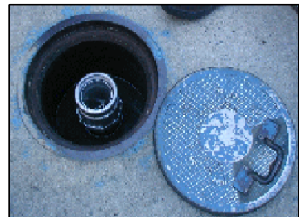
Sample Spill Protection
