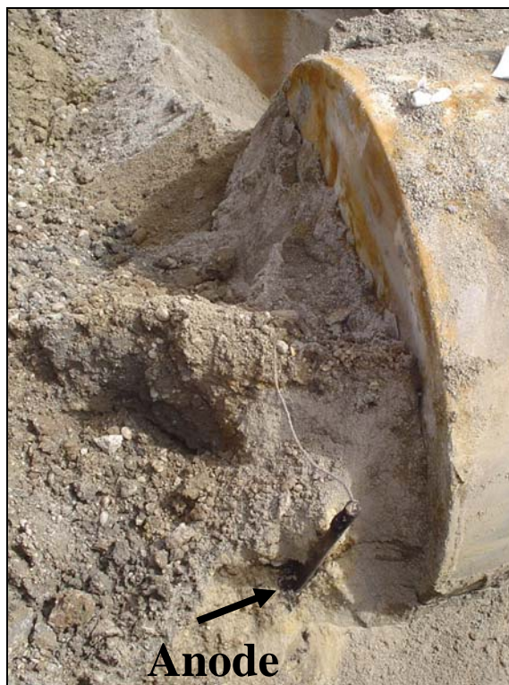
Half buried Metal Tank with Impressed Current Anode
