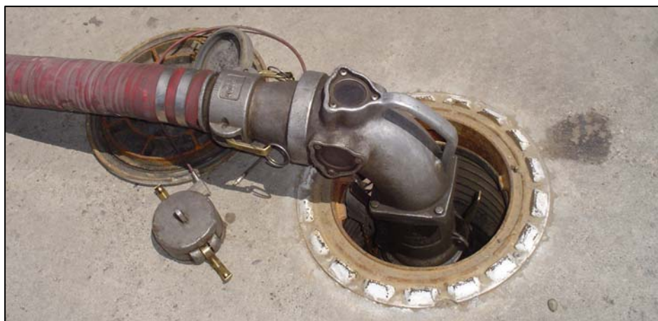
Delivery Hose Connected to a Fill Riser
