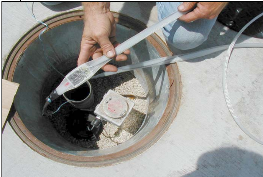
Sensor for Interstitial Monitoring of Double Walled Tanks
