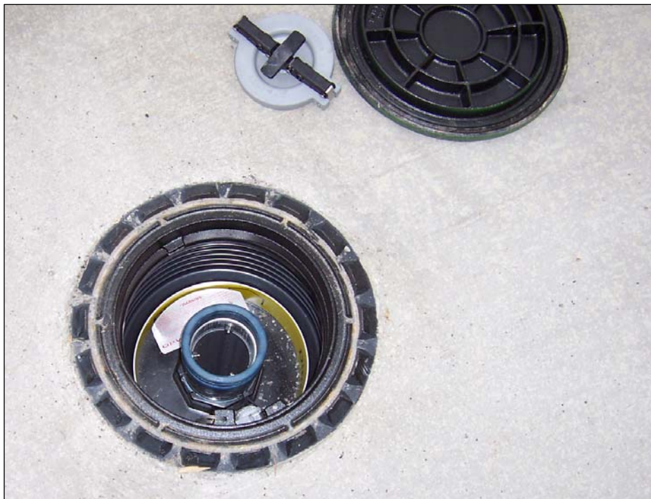
Spill Bucket and Fill riser with cap off
