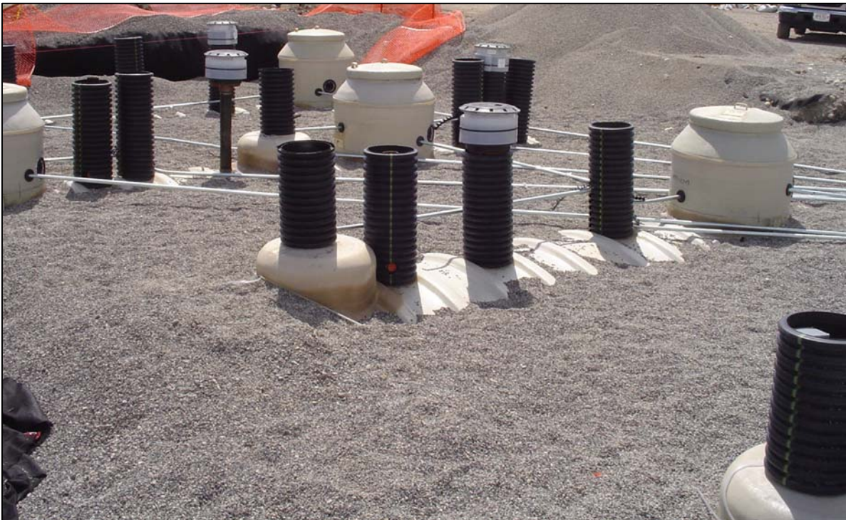
New Tanks and Risers Partially Buried in Pea Gravel
