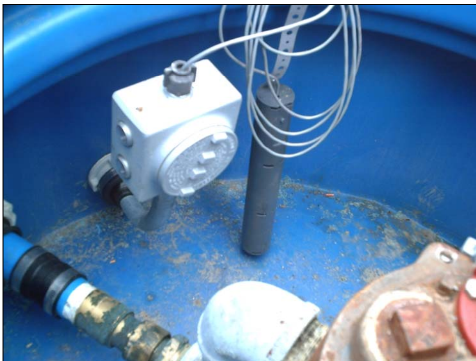
Sump used to monitor interstitial monitoring (Notice the sump sensor near the bottom of the sump and the black boot on the piping is pulled back to allow product to drain into the sump)
