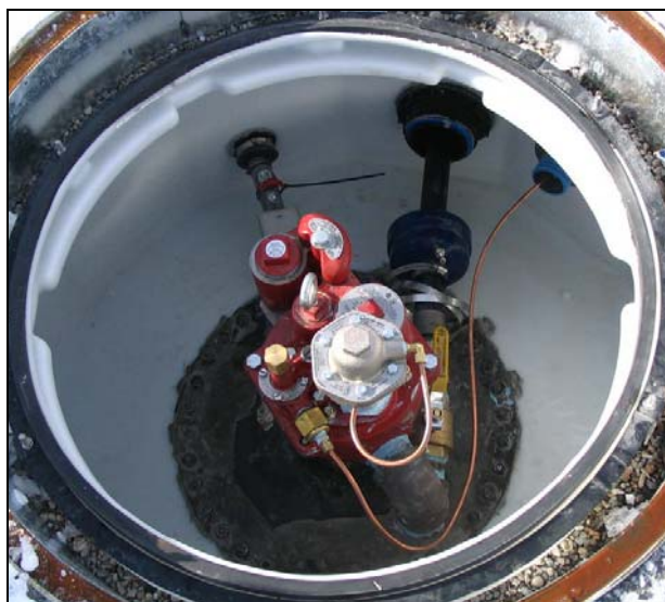
Containment Sump of a Pressurized System
