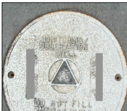
Sample Monitoring Well Cover
