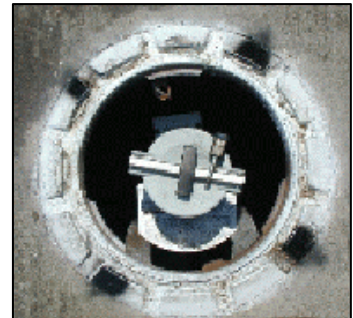
Sample Spill Protection
