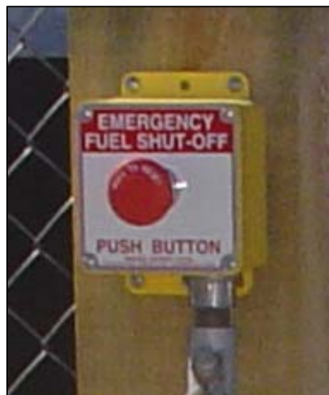
Emergency Shut-Off Switch
