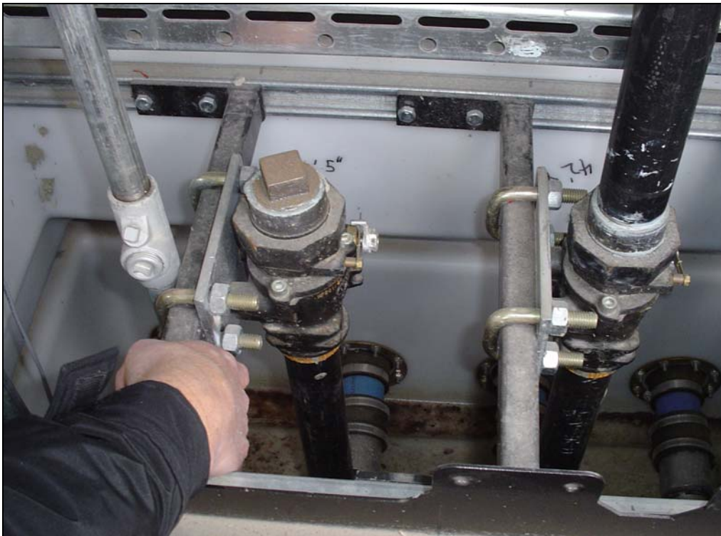
Sufficiently Anchored Shear Valves Under A Dispenser
