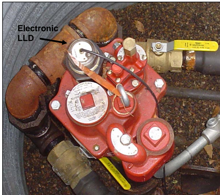
Electronic LLD installed on a STP
