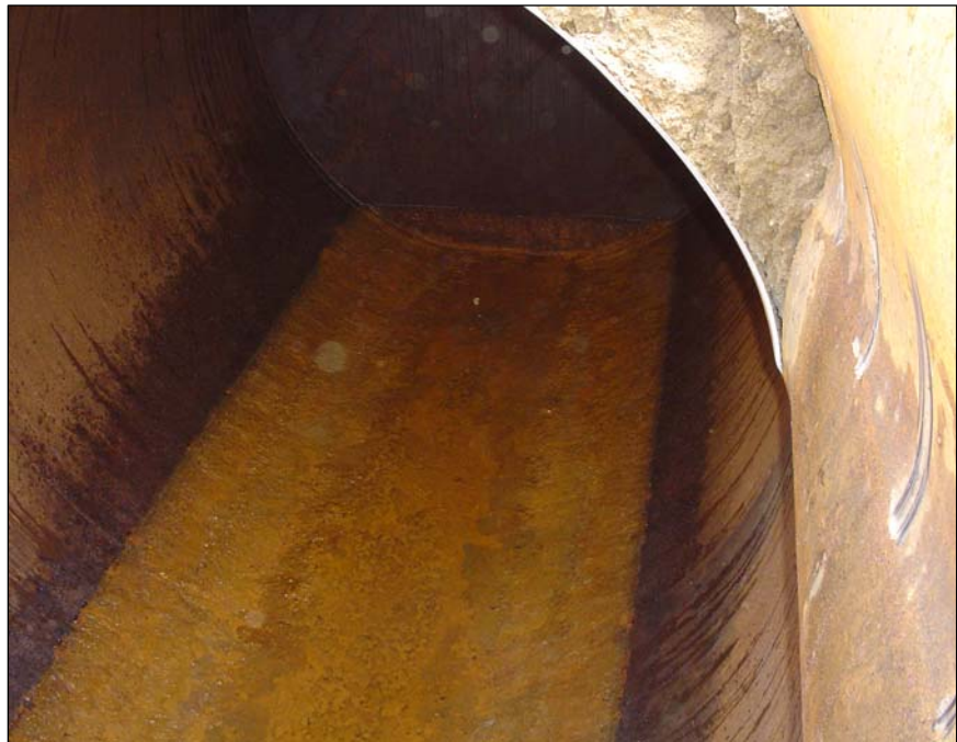
Bad Corrosion Due to Water in the Tank
