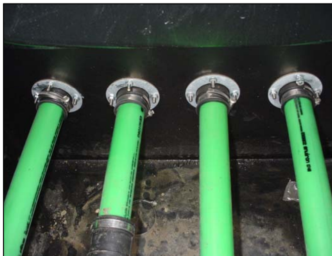
Sample Flexible Piping In A Sump
