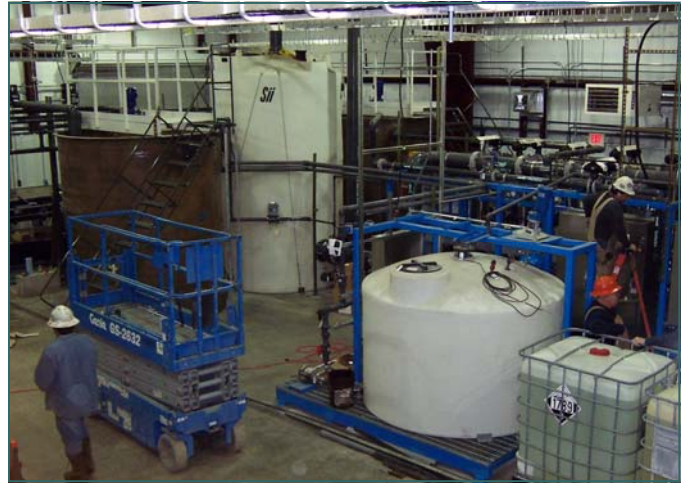
New state-of-the-art water treatment plant..
