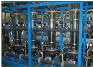
Water filtration system treats an average of 91,000 gallons a day.
