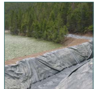
Beartrap Creek diversion around Mike Horse Dam.
