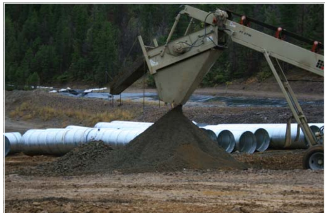
Materials being screened to ascertain suitable, non-leaking core for dam
