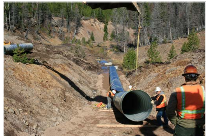
New drainage pipes being laid
