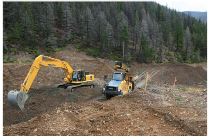
Construction begins at location of new drain system
