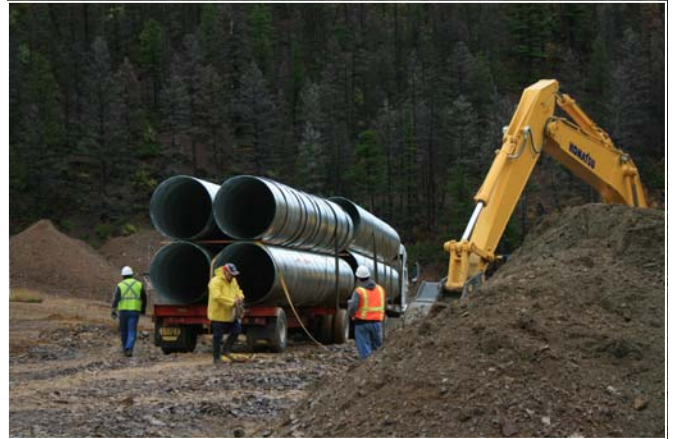
New drain pipe arriving at site
