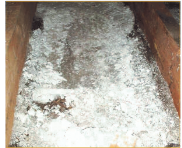
Karstolite insulation in an attic
