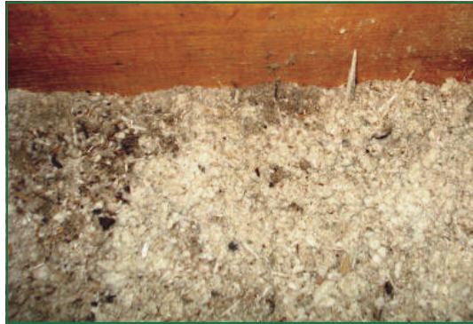
Karstolite insulation in an attic
