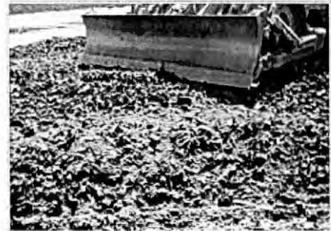
Shredded scrap tires used as road base in Odessa, Texas.
