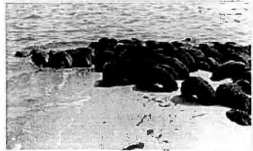
The Army Corps of Engineers used tires to protect marshland on Gaillard Island, Alabama from wave action, enabling plant root systems to establish.
