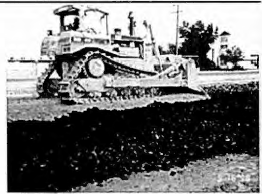
Road embankment constructed with shredded tires in El Paso, Texas.
