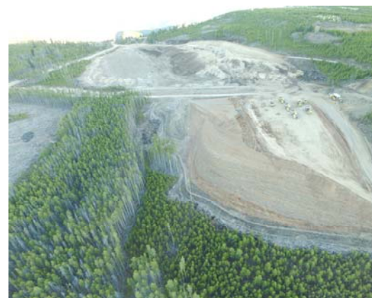
An aerial view of the repository area, where approximately 400,000 cubic yards of contaminated tailings and waste rock are now stored.
