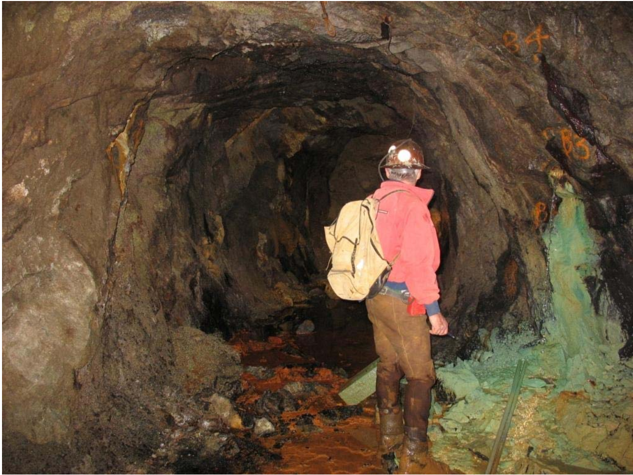
Photo 3-13. Oriole Adit exploration drill hole seep, malachite on rib, and ferricrete on sill.
