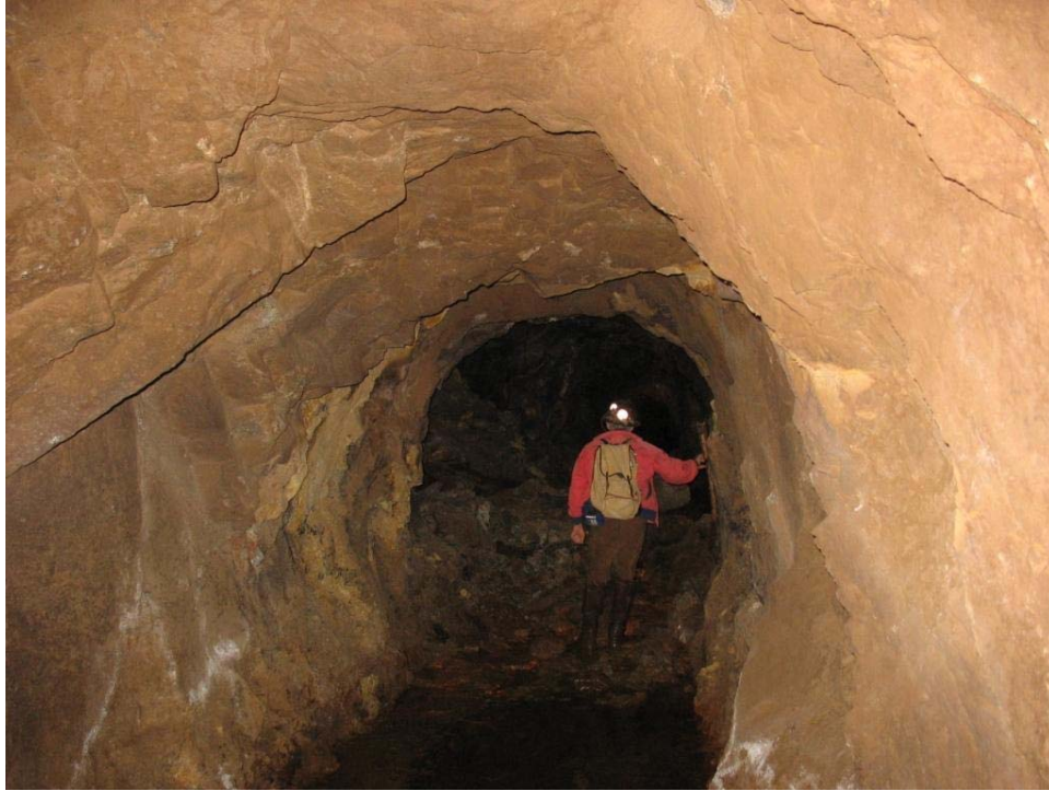
Photo 3-9. Oriole Adit (1,070 feet).
