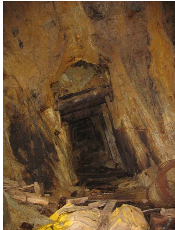
Photo 3-11. Oriole Adit cross-cut drifts.
