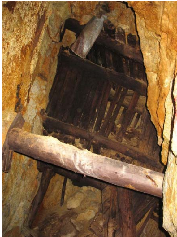
Photo 3-12. Oriole Adit stop.
