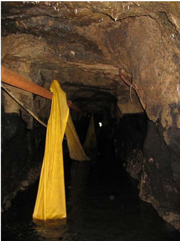
Photo 3-10. Oriole Adit utilities.
