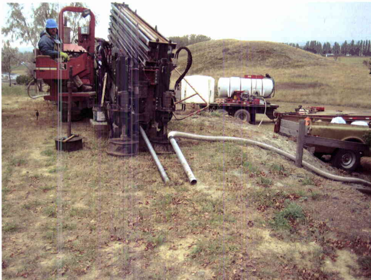
Advancing HDD Hole Number 1
