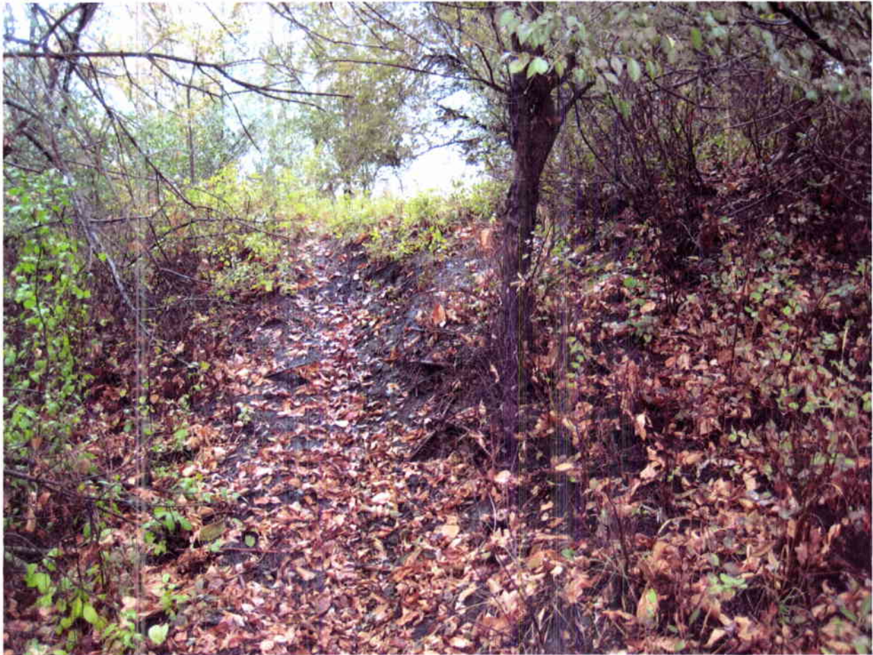
Slack pile at collapsed Adit 2
