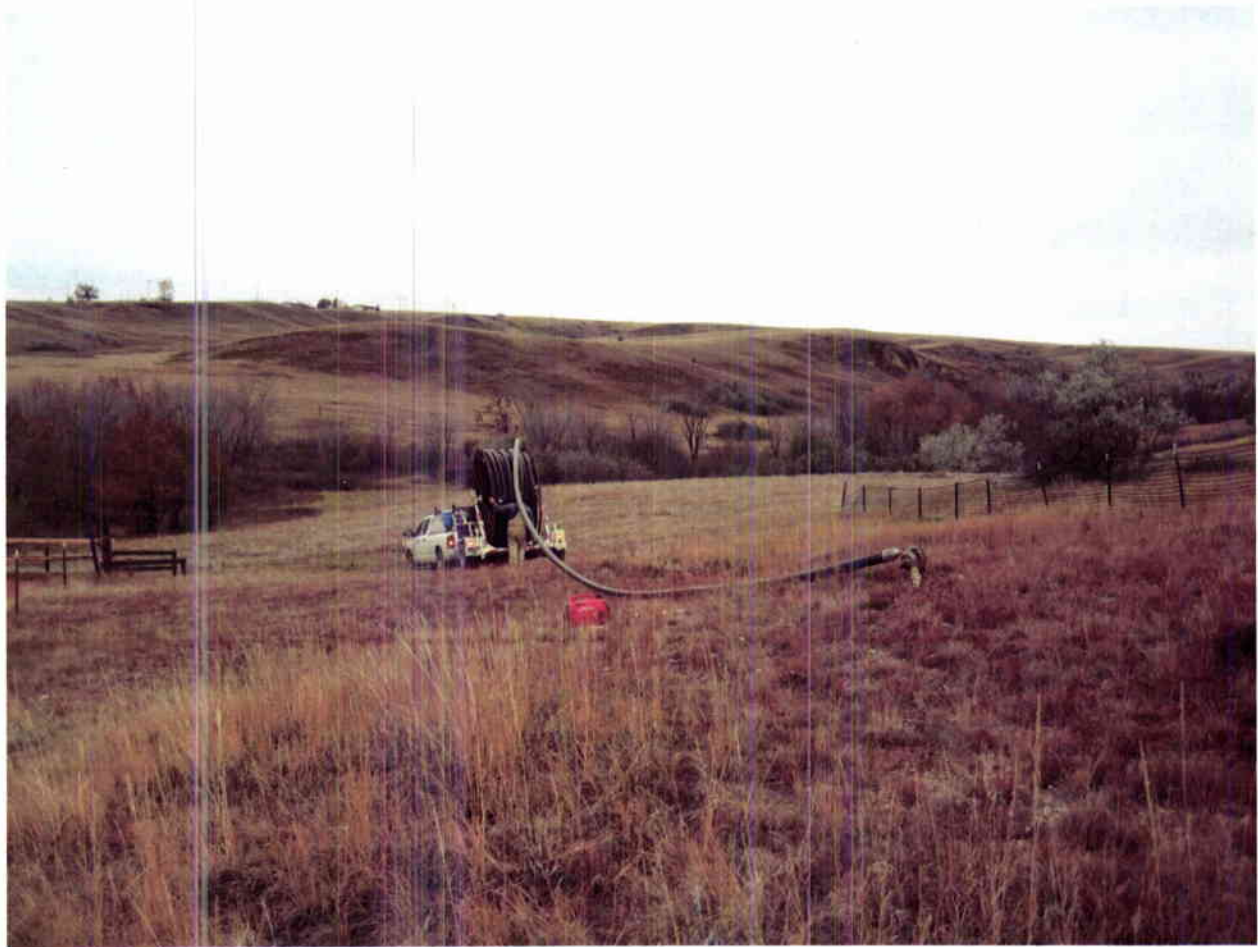
Pulling HDPE Pipe Back Through Borehole
