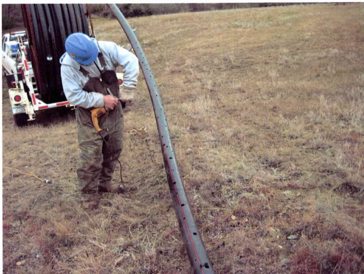
Perforating HDPE pipe for grout injection
