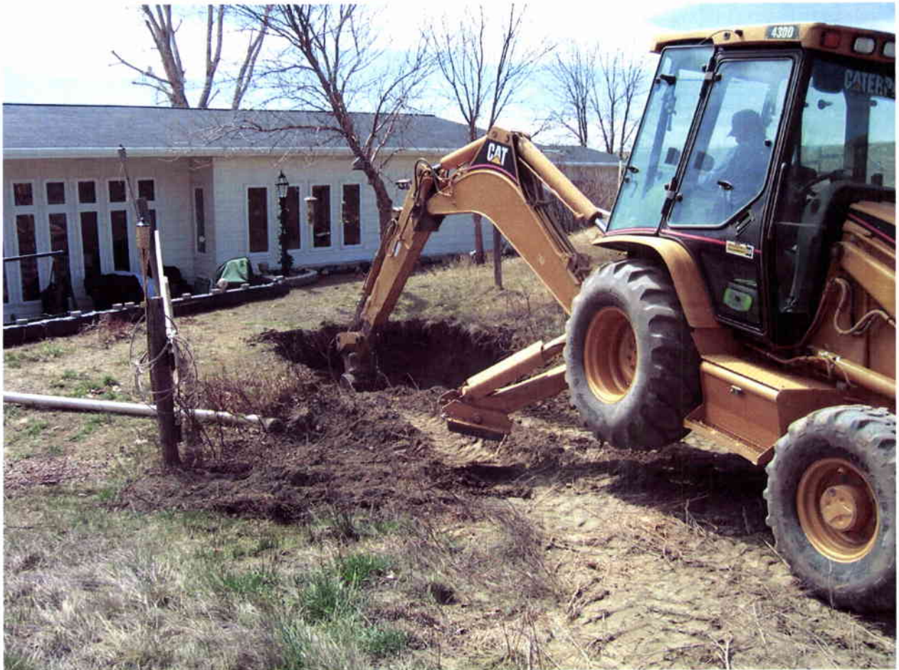
Over-excavating and backfilling Subsidence Feature 1
