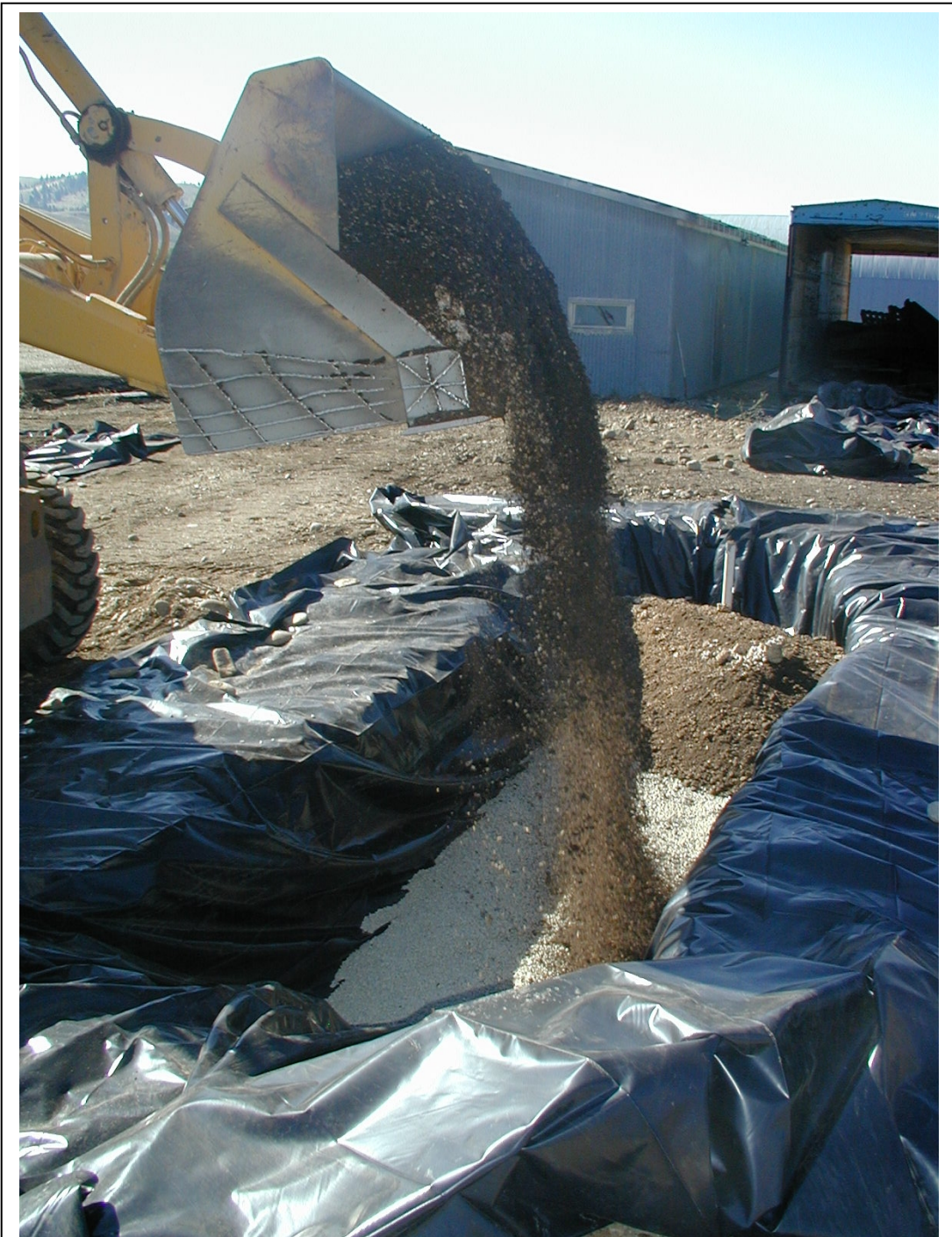
Figure 11. Loading inoculated soil into the biocell.
