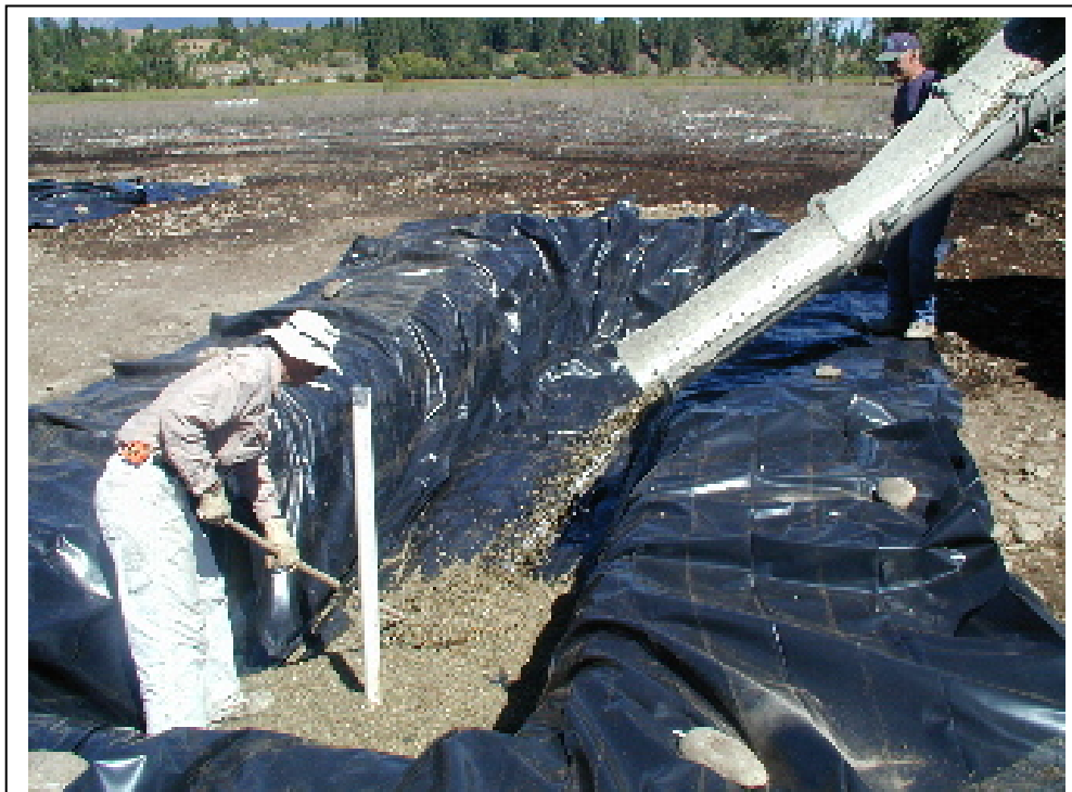
Figure 7. Pea gravel being loaded into the lined excavation.
