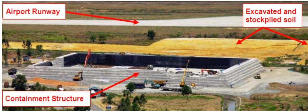
Pile containment structure
