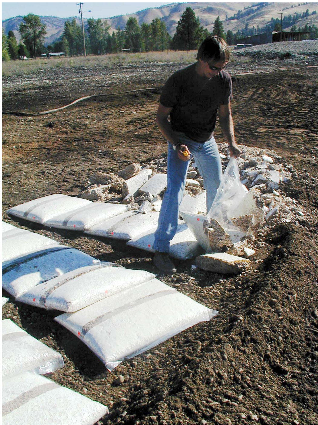
Figure 9. Opening the bags of fungal pelleted inoculum on top of the soil to be mixed and treated.
