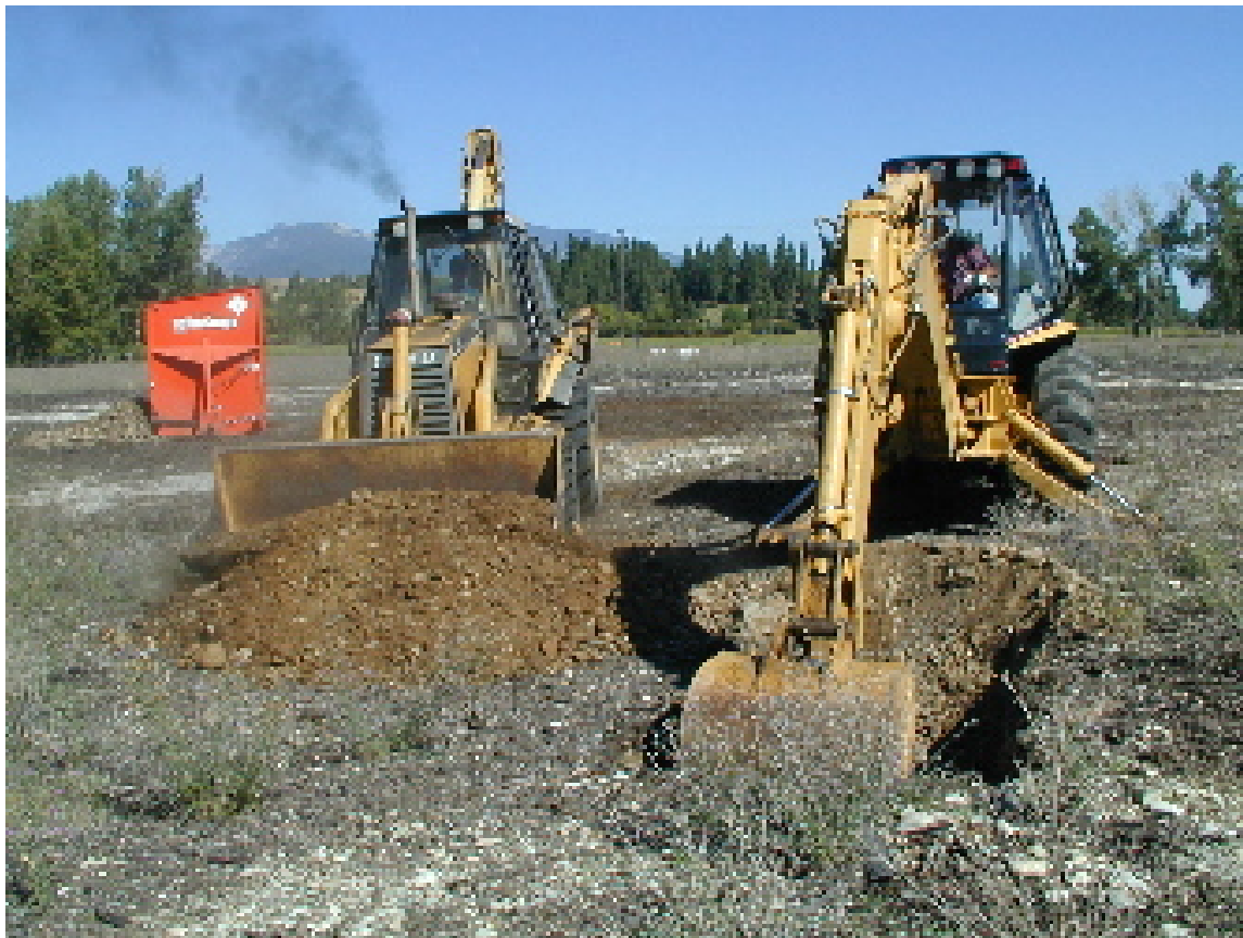
Figure 6. Excavating soil for use in the biopiles.
