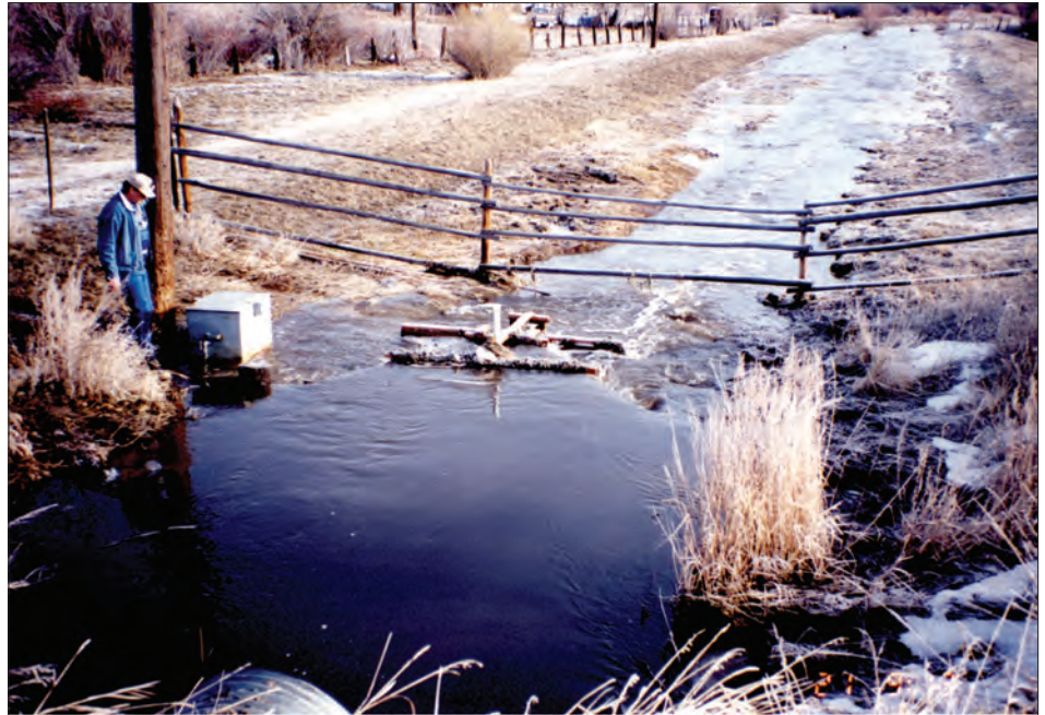
Figure 3. Grove Gulch streamflow at Rowe Road during a large run-off event in 1995. Picture taken at the gauging station on the south side of Rowe Road shows streamflows overtopping the weir. Historically (pre-1982), large sediment loads were transported into Blacktail Creek during similar events.
