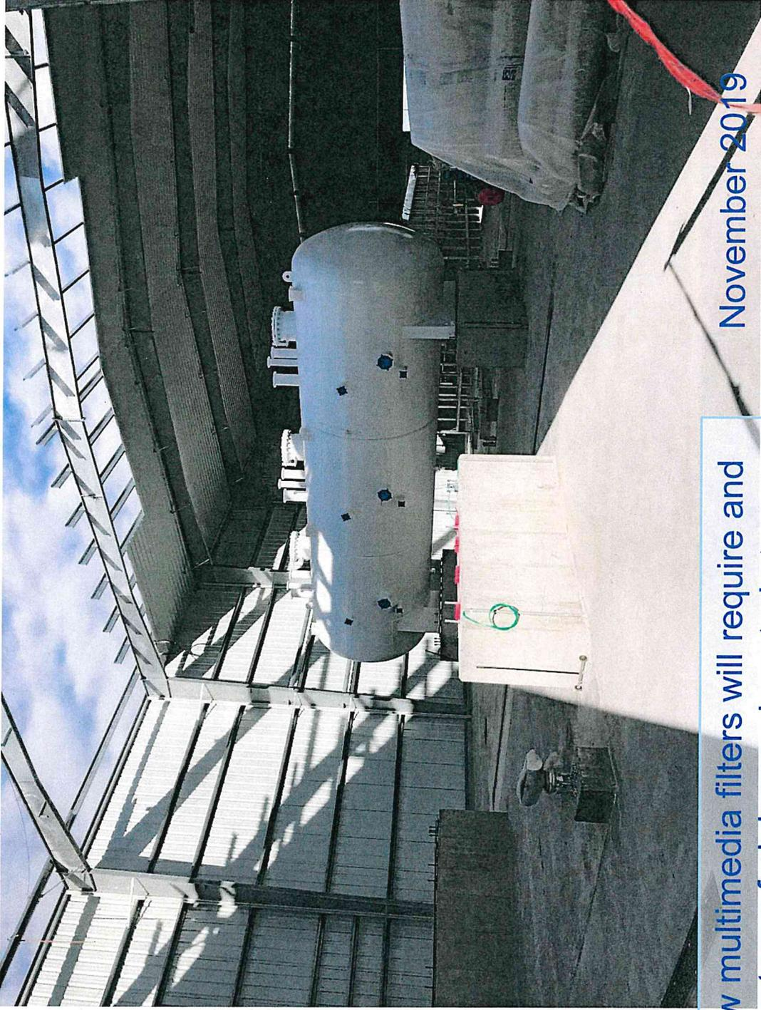
The two new multimedia filters will require and extensive system of piping and controls to enable efficient and effective backwashing.
