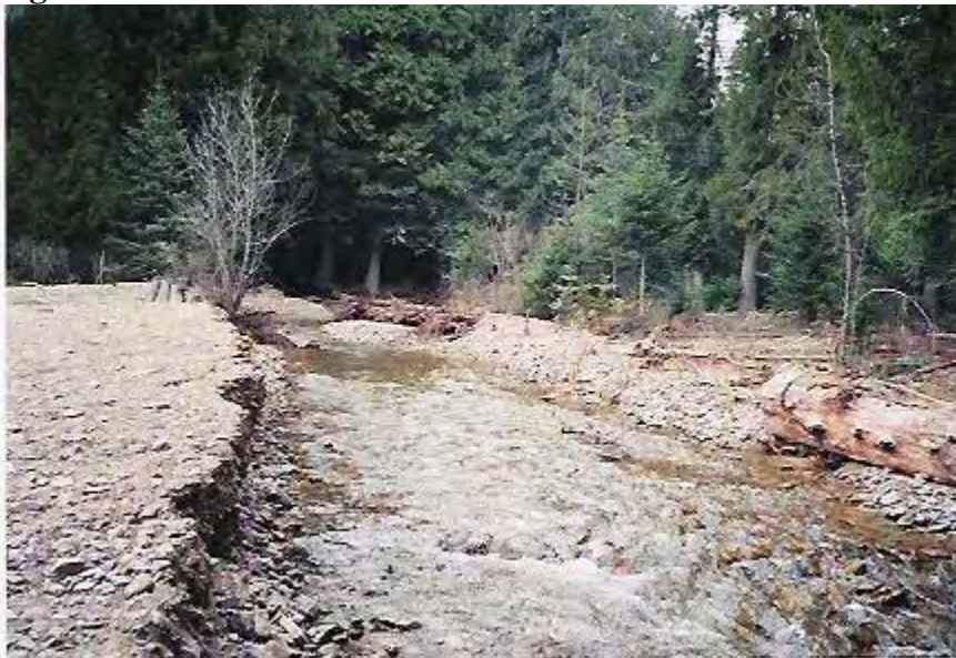
Figure 4-4. Area of Unstable Stream Reach.
