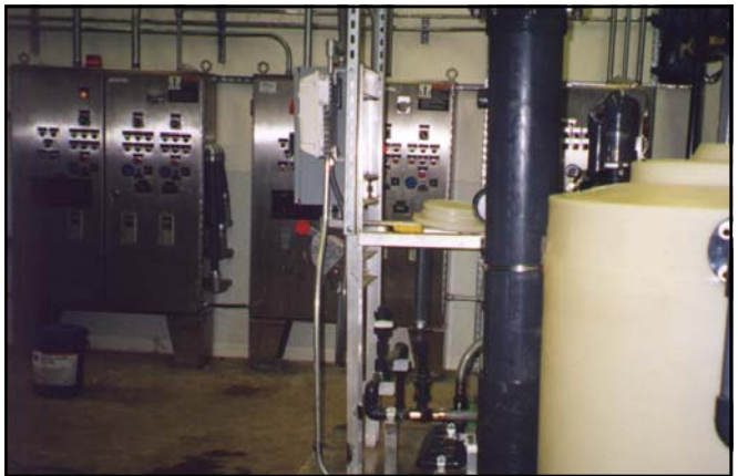
Plant treats 345 gallons per minute. (Photo property of DEQ)
