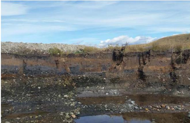
*Contaminated material in one of the streambanks in Phase 2. This material was removed and disposed of at the regional repository.*
