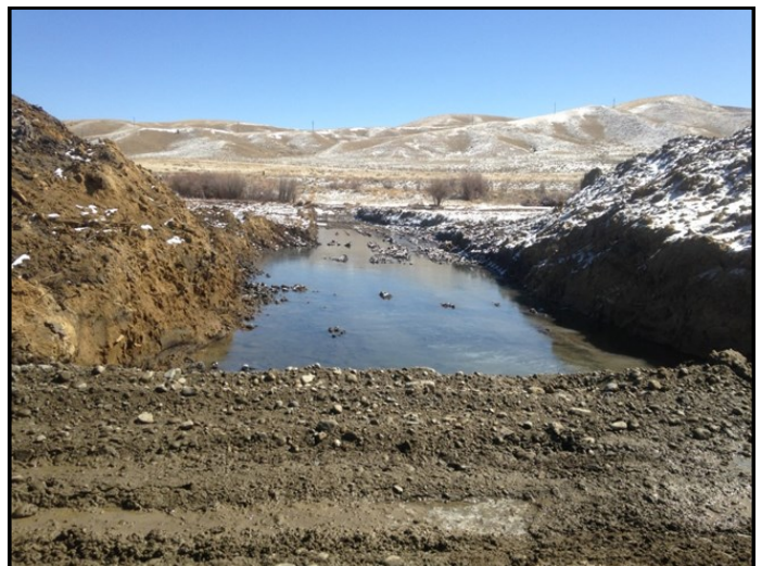
Excavations such as dewatering trenches present hazards to people walking across the site even when equipment is not present. These trenches can be slippery and have unknown depths as well as unstable banks.
