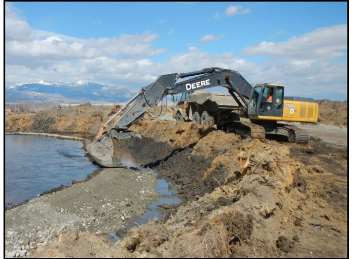
Excavators removing tailings from the banks of the Clark Fork present a hazard to floaters. Large equipment operators have limited visibility and may not see people within reach of the swinging excavator arm.
