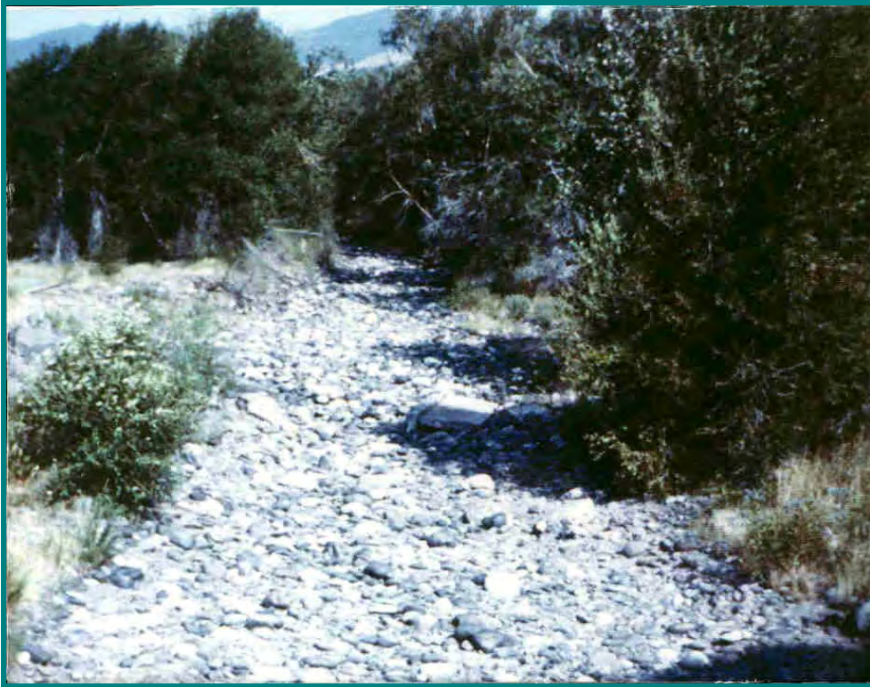
BEFORE (Prior to 1998) Photo by FWP
