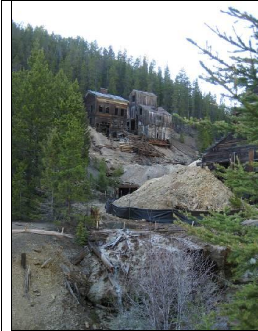
Figure 5-3a. Galena Creek Mine Adit & Mine Wastes
