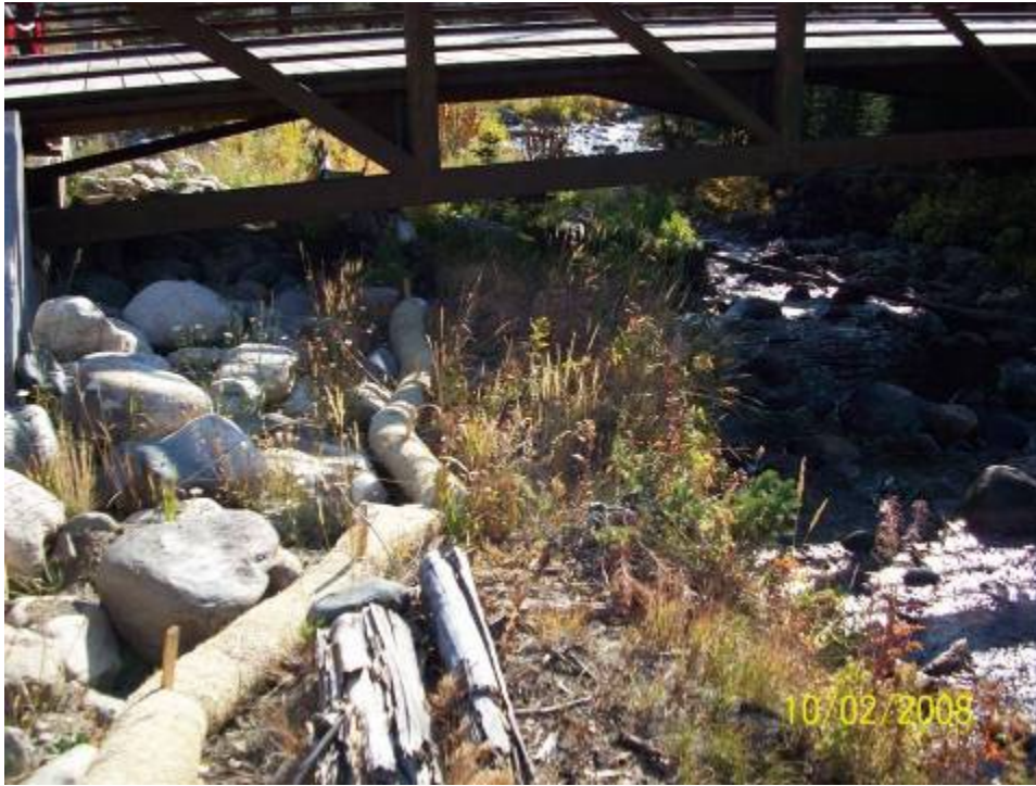
Photo 1. Fiber wattles used at a road crossing.
