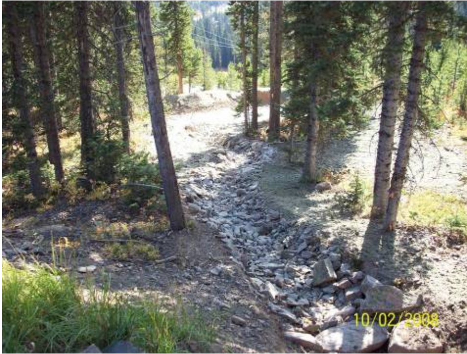
Photo 3. Rock lined storm water conveyance channel.
