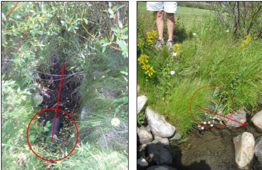
Figure 6-25. Cross-drain discharges to the West Fork Gallatin River
